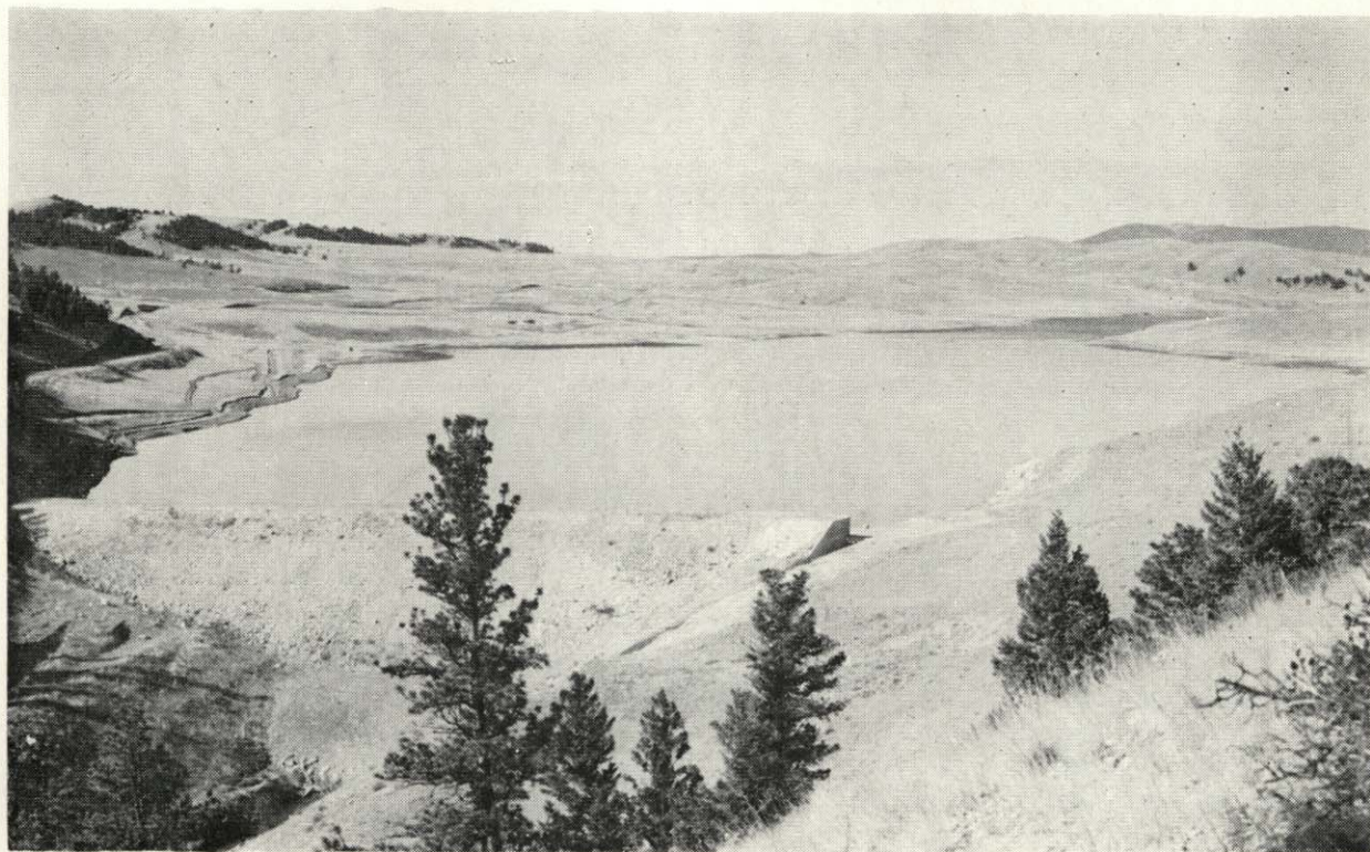
DURAND DAM AND RESERVOIR: A portion of the State Water Conservation Board's Upper Musselshell Project on the North Fork of the Musselshell River. The photograph shows the dam with its spillway (right) and outlet (bottom), and the reservoir as it was in October, 1950.
