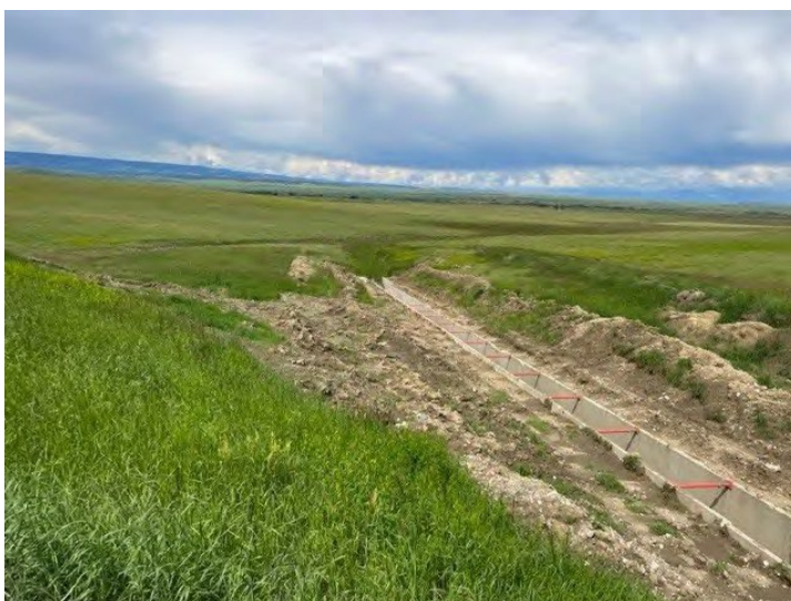
Spillway Chute at East Dam
