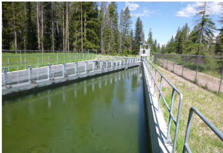
Main Canal Vertical Panel Fish Screen
