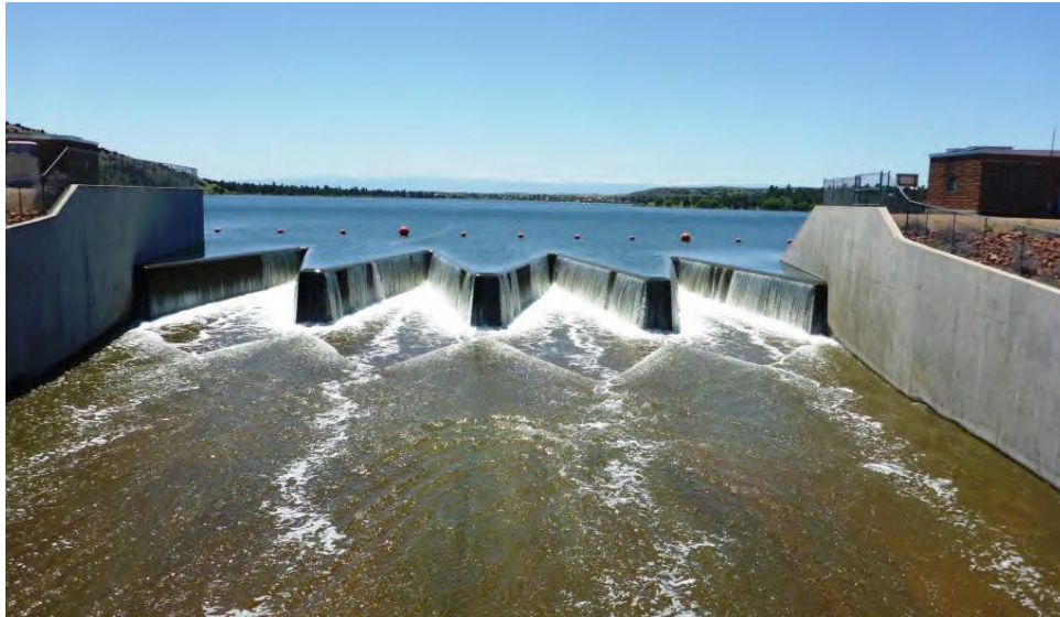
Labyrinth weir at top of spillway
