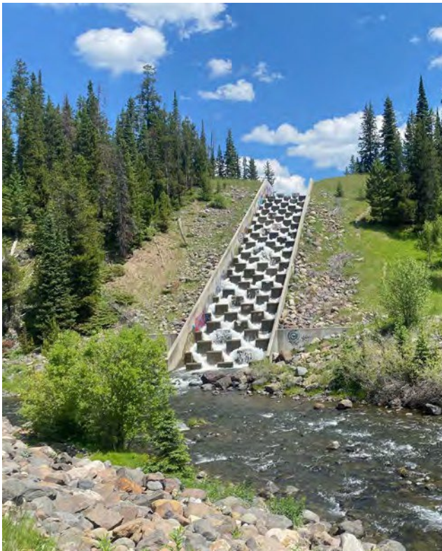
Lower spillway baffled drop
