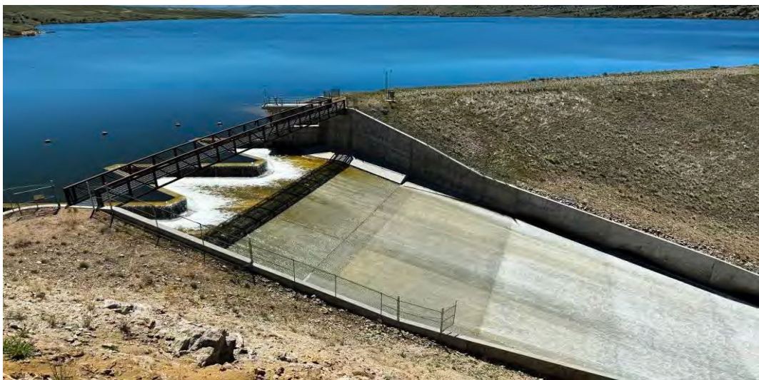
Labyrinth weir spillway and footbridge
