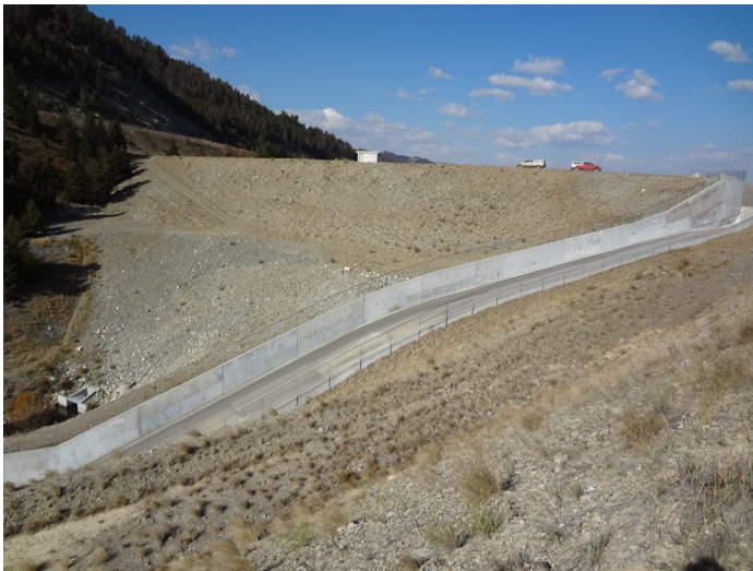
Spillway and Gatehouse
