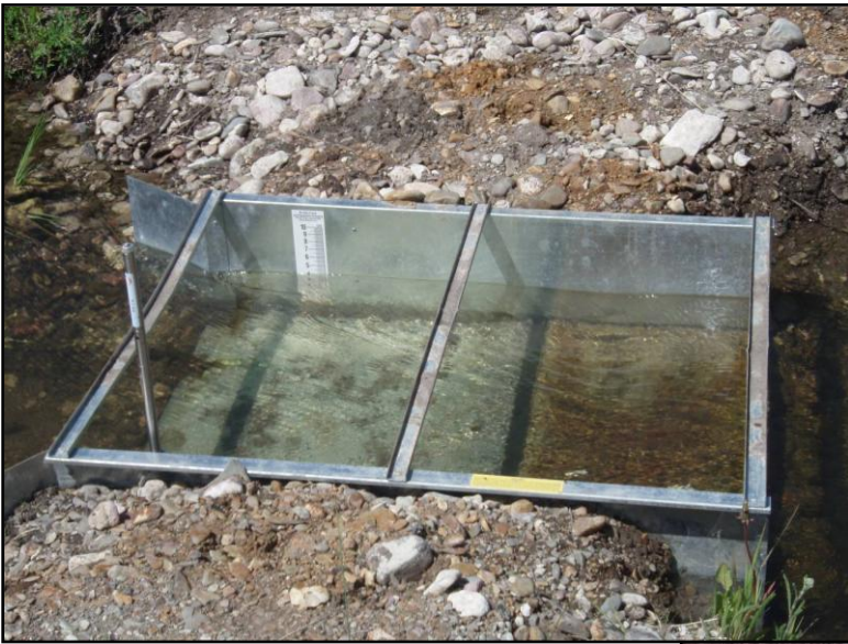
Photos 3 and 4. Flumes on the Peterson and Reeverts surface irrigation systems.
