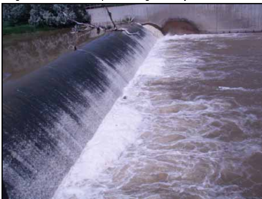
Figure 2.12: Fort Belknap Indian Irrigation Project Diversion Dam.
