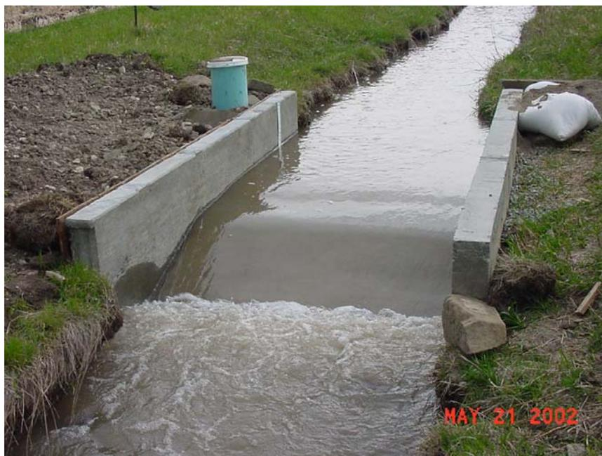
Photo 3. Ramp flume that was installed on the Lower Big Ditch.
