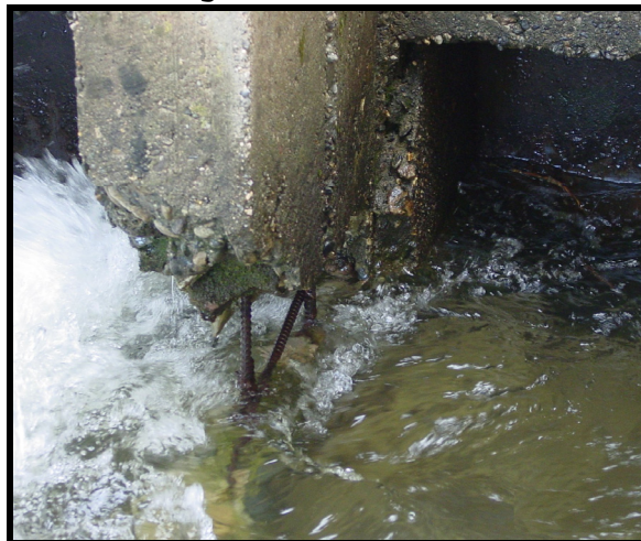
Photo 10. Damage to the Concrete on the Headgate.
