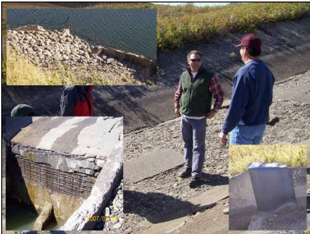
Photo 8.8 – Damage and Wear to the U.S. St. Mary Canal Drop Structures. Photo: John Sanders
