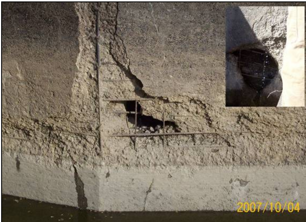
Photo 8.9 – Damage and Wear to the U.S. St. Mary Canal Drop Structures.
