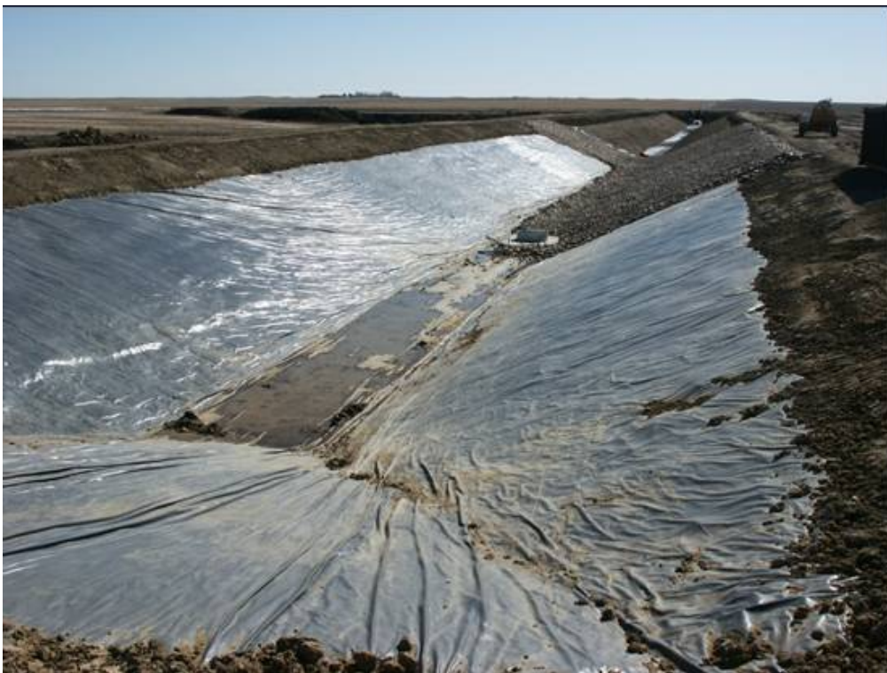
Photo 8.39 – Irrigation Canal with Poly and Gravel Armour Lining.
