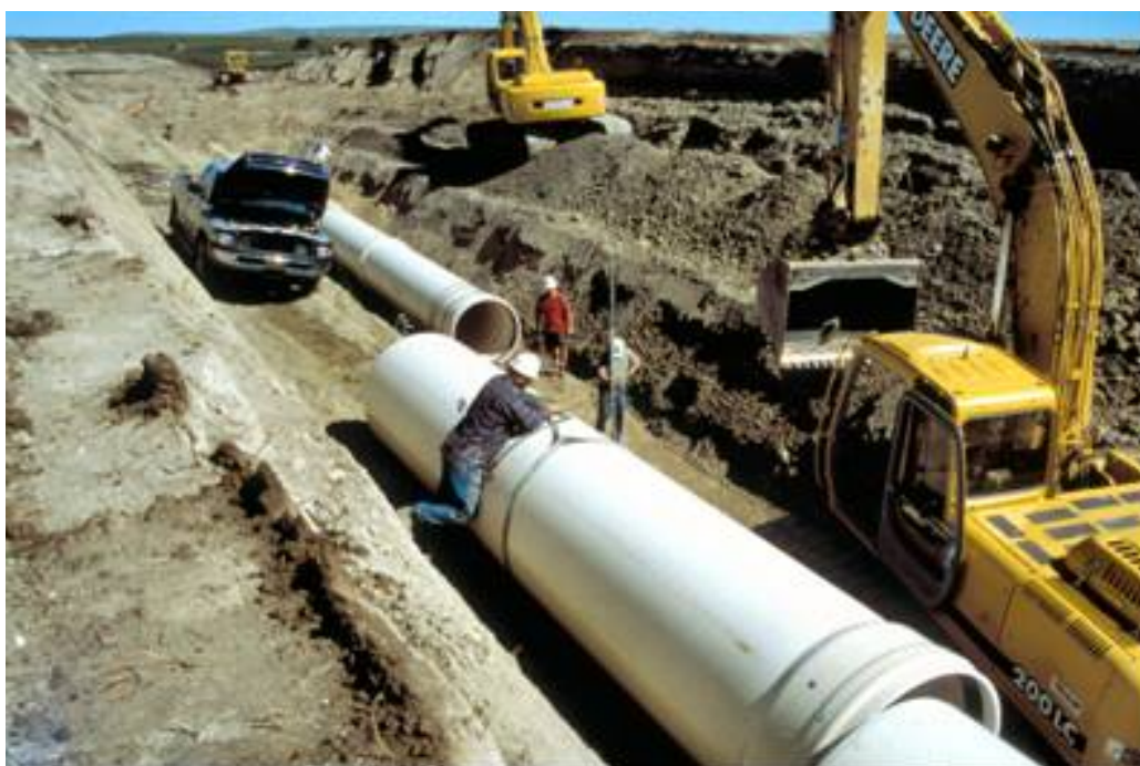
Photo 8.37 – Irrigation Pipeline Installation. Photo: Alberta Agriculture and Rural Development
