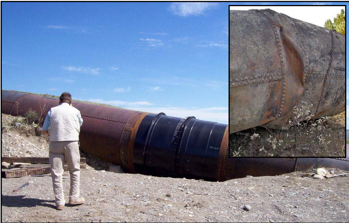
Photo 10.2 – Showing infrastructure deterioration at the canal siphon. Photo: John Sanders
