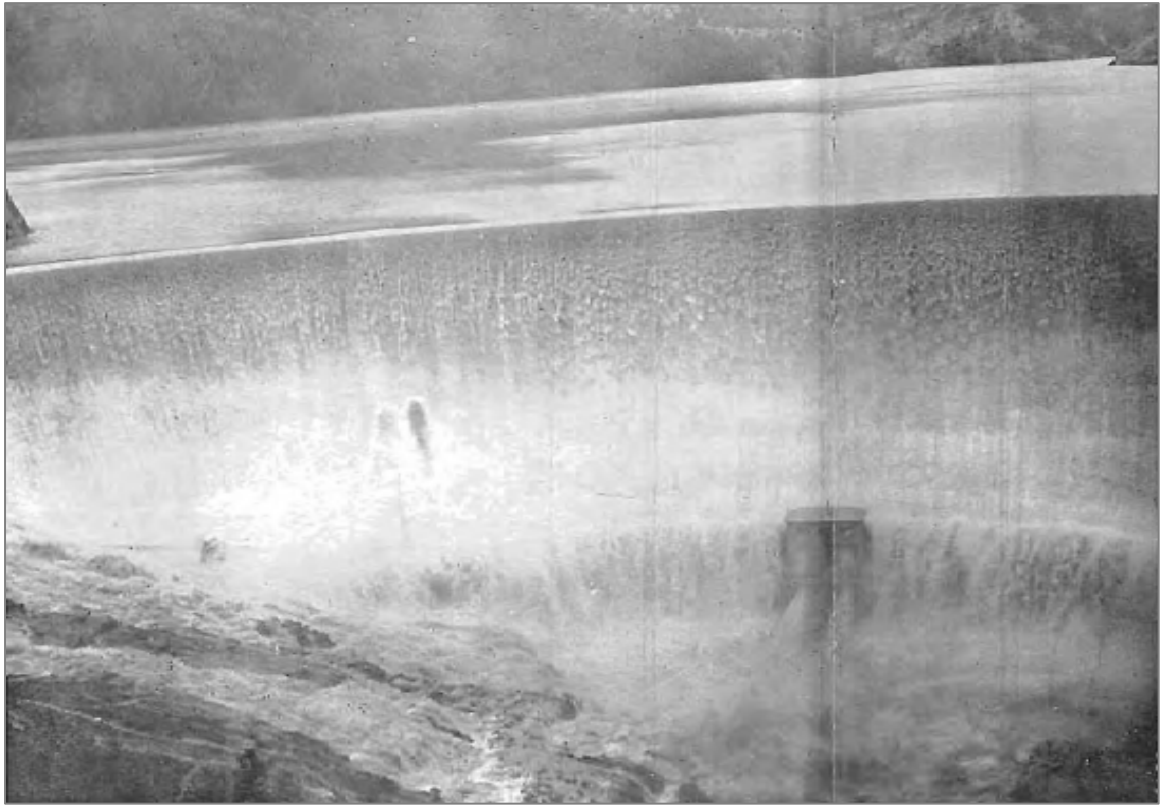
Figure 1-2. 1964 Flood Overtopping Gibson Dam (adapted from "Montana Flood 1964" published by Great Falls Tribune-Leader).
