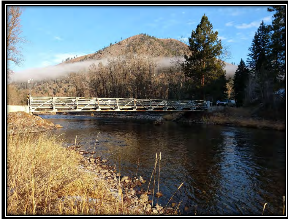
Photograph 1: Rock Creek – Stage Station Road at RS 1,666 (S141)
