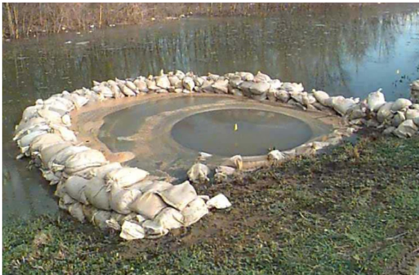
Figure 20: Sandbag Ring Levee around a Boil at the Downstream Toe of an Embankment Dam
