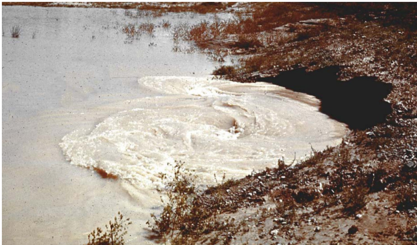
Figure 7: Photo of a Whirlpool at the Upstream Slope of an Embankment Dam
