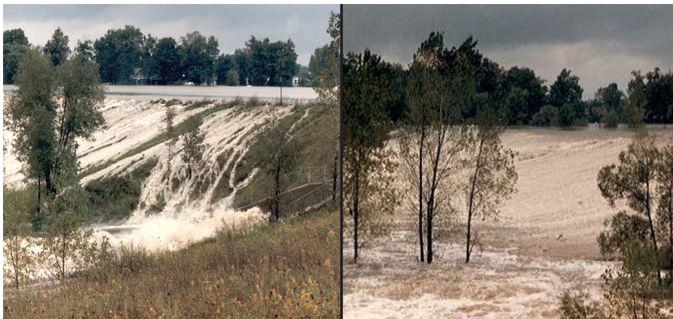
Figure 4: Examples of Dam Overtopping During a Flood
