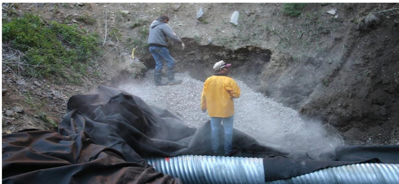
Figure 26: Example of Filter Diaphragm Construction around a Conduit in an Embankment Dam
