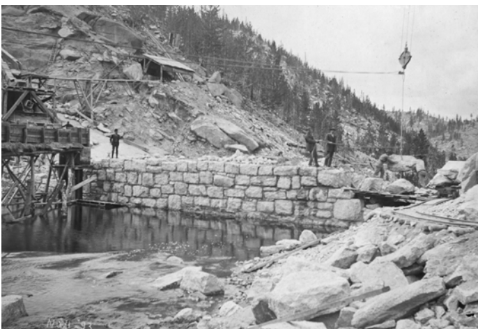
Basin Creek Dam under construction & upon completion (1893 to 1913, Butte, Montana). Photo Courtesy of City/County of Butte Silver Bow
