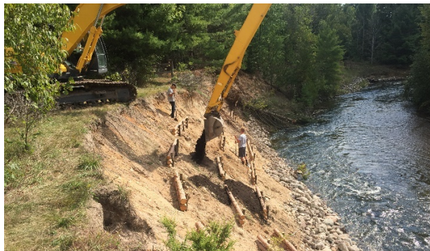
Figure 3: Reinforced logs are being used to stabilize a sluffing riverbank.
