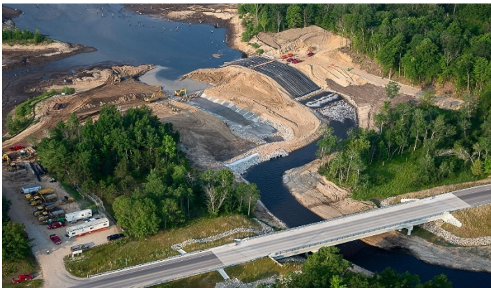
Figure 6: Dam removal in process utilizing multi-stage siphon and spillway dewatering system.
