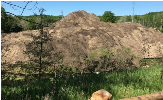
Figure 8: Sediment spoils pile mid-construction.
