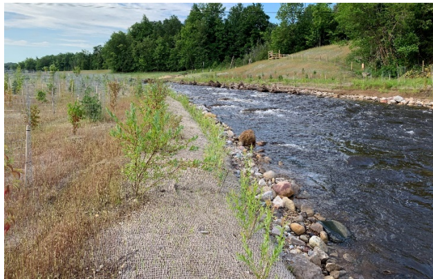
Figure 2: Soil encapsulated channel banks with live stakes installed along the bank and floodplain bench are utilized to stabilize the stream banks.
