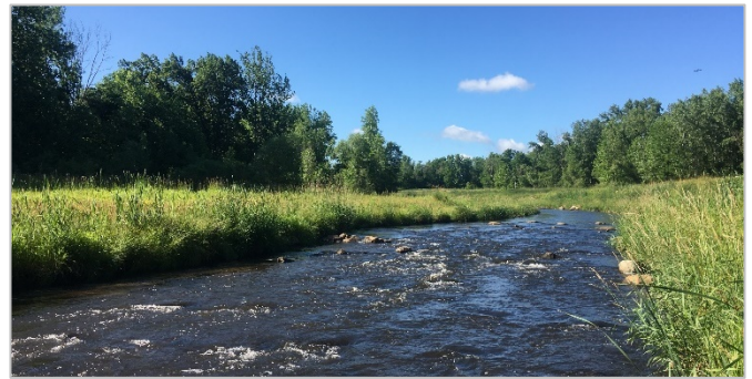
Figure 5: Engineered riffle with rock boulders to provide grade control on impounded sediment and design to allow fish passage.
