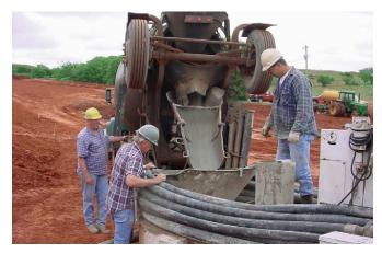
Figure 7. Grout being delivered to the pumping truck. [1]
