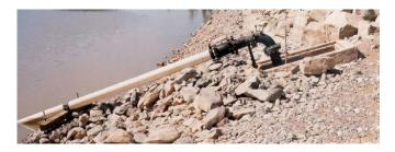
Figure 3. Siphon used to lower the reservoir water surface through the upper entrance of an outlet works intake structure. [1]
