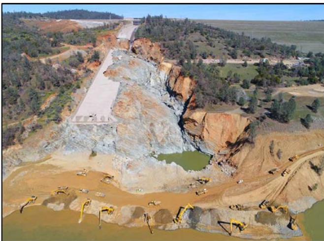
Figure 1. Final Damage at the Oroville Dam Service Spillway [1].
