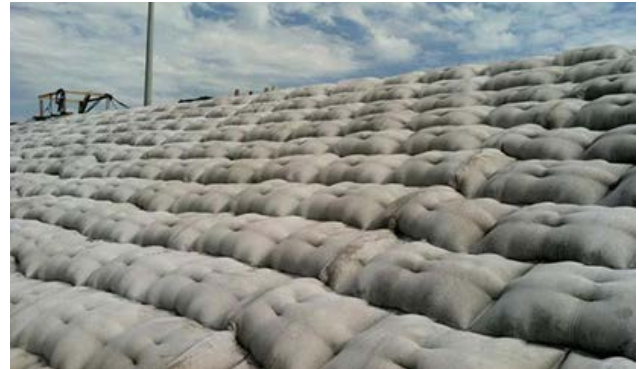
Figure 5. Fabric-Formed Articulating Block Mats (Courtesy of Synthetex).
