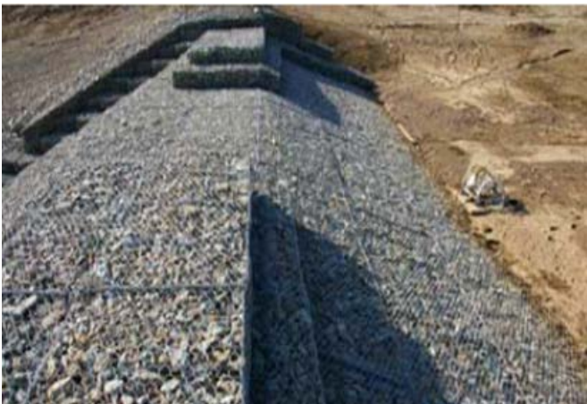
Figure 3. Gabion Installation on a Slope [1].
