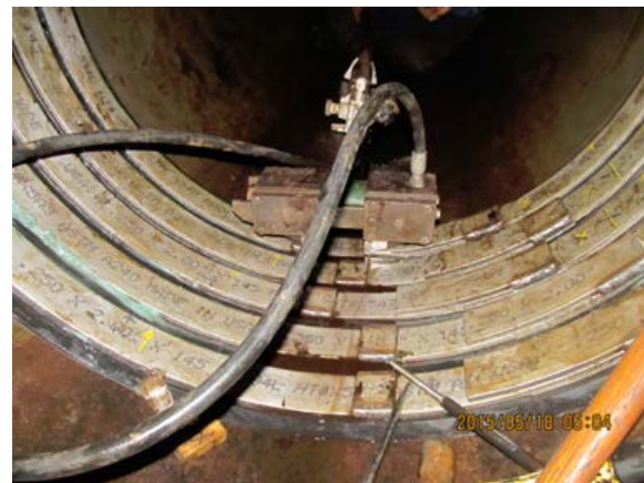
Figure 9. Retaining Compression Bands Locked into Place by a Hydraulic Expander (photo courtesy of NRCS).
