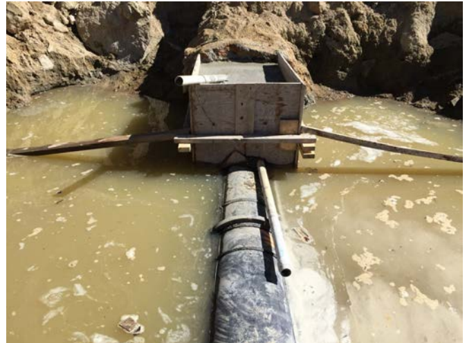
Figure 3. Cellular Grout Placement at Estler Lake Dam
