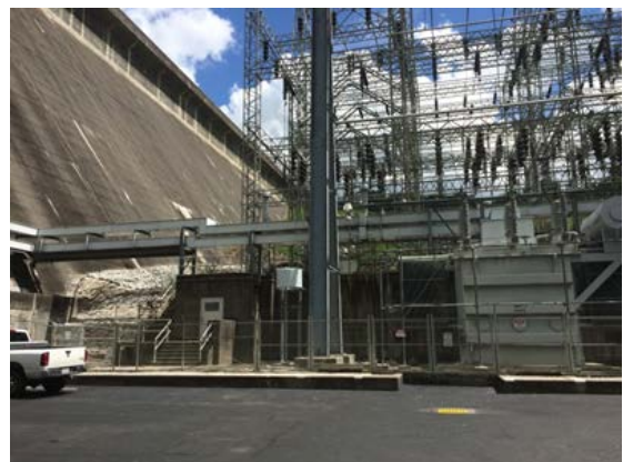
Figure 3. Dam and switchyard where EMI could interfere with UAS operation.
