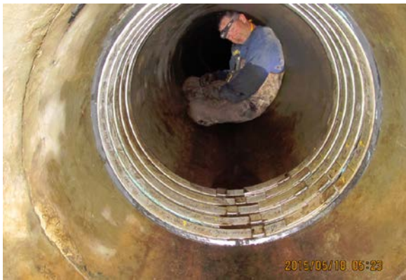
Figure 10. Mechanical Seal and Completely Installed (photo courtesy of NRCS)
