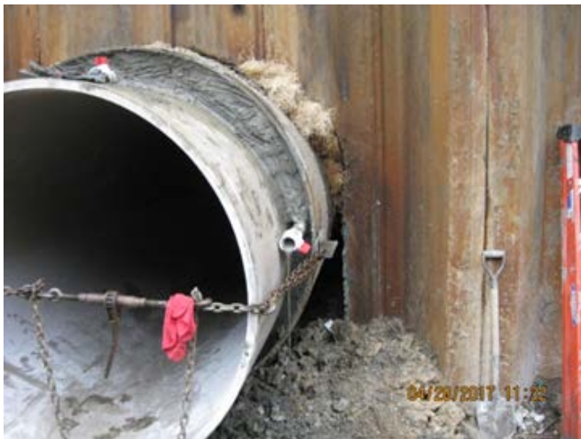
Figure 1. Annular Space Slipline Grouting with Cellular Grout
