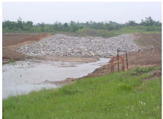
Figure 4. Riprap Installation [1].
