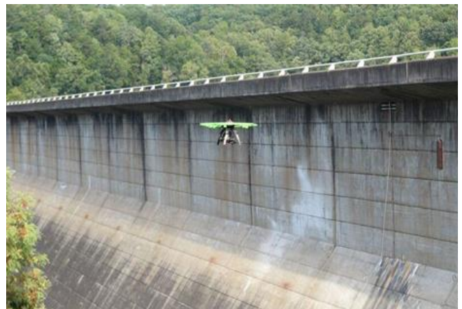
Figure 1. Employing UAS to Inspect a Concrete Dam
