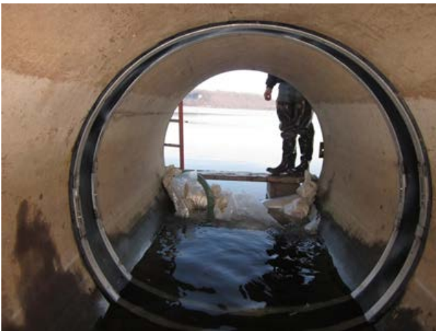
Figure 4. Example of a Circular Mechanical Rubber Seal in a Concrete Conduit (photo courtesy of HydraTech)
