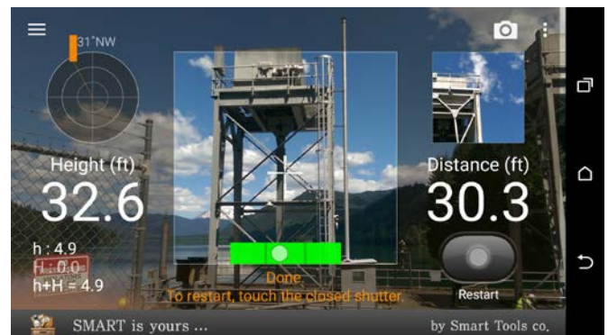
Figure 3 – Measuring Height of Intake Tower with Smart Measure Pro
