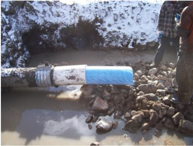
Figure 8 – CIPP after Installation
