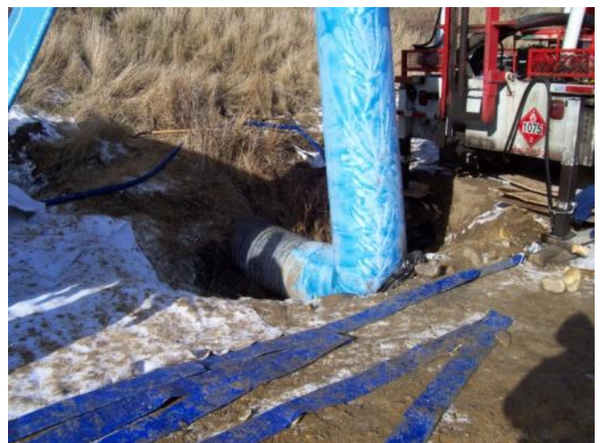
Figure 7 – CIPP Being Installed to Rehabilitate 24-inch CMP
