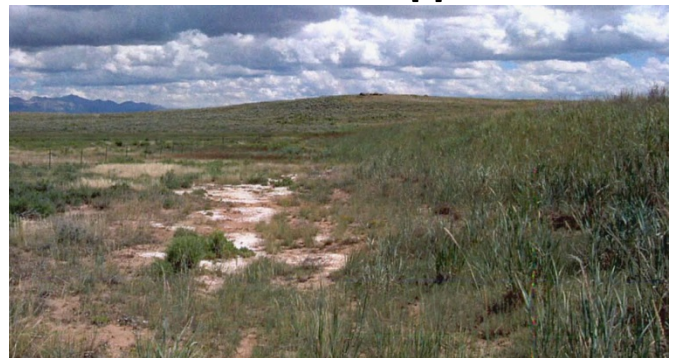
Figure 9. Surface Staining from Intermittent Underseepage at a Colorado Dam
