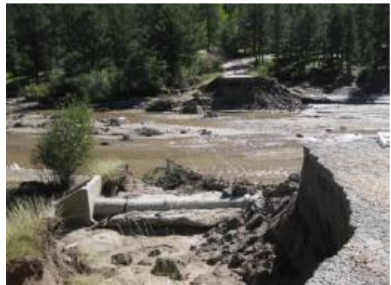
Photo 7: Rainbow Lake Dam post-failure looking across from left abutment.
