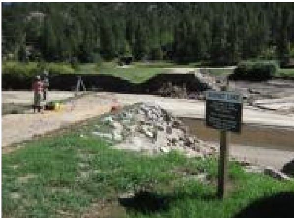
Photo 5: Sunset Lake Dam post-failure looking across and downstream from left abutment.
