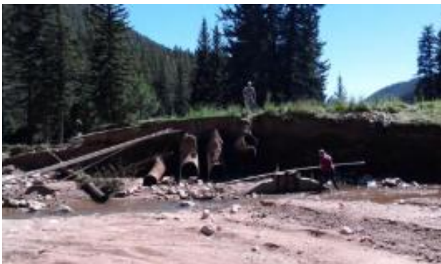
Photo 2: UEV Dam post-failure looking upstream.
