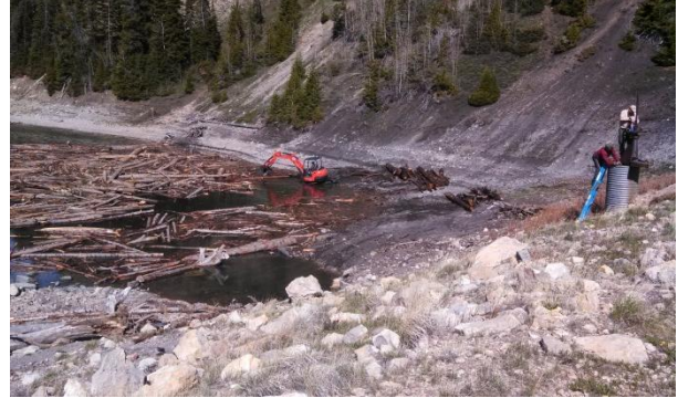
Photo 5. Reservoir Debris at Intake during a Period of Reservoir Drawdown. Photo by Wyoming State Engineer's Office
