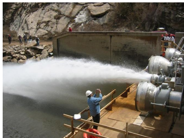
Photo 2. Outlet Commissioning Test. Photo from the Dam Safety Branch of the Colorado State Engineer's Office.
