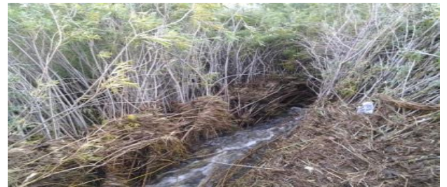
Photo 16: 2-foot-wide notch formed in CH1 Dam spillway.
