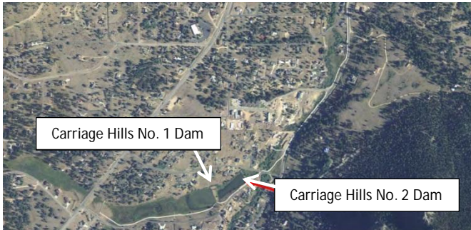
Photo 11: Aerial image of CH1 and CH2 Dams.
