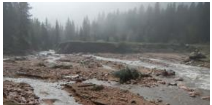
Photo 3: LEV Dam post-failure looking upstream.
