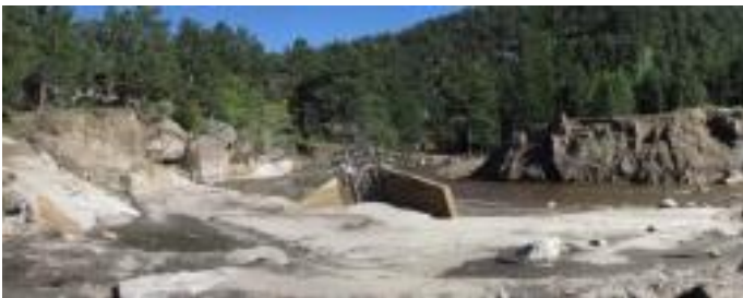
Photo 10: Meadow Lake Dam post-failure looking downstream from within reservoir.
