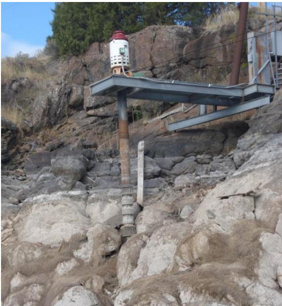
Photo 4. Irrigation Well Left High and Dry by Reservoir Drawdown Increased amounts of debris may be produced from the newly exposed rim, which can begin to clog spillways and trashracks. For large volume releases, the increased energy in the reservoir can transport previously stable sediments in upper reaches of the
