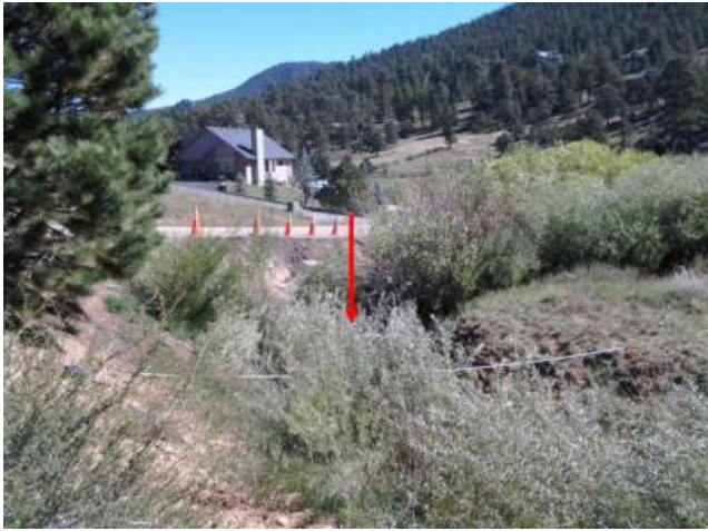
Photo 13: CH2 Dam spillway looking downstream. Note heavy vegetation in spillway.
