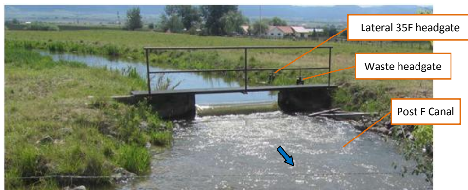
Figure 52. Existing check structure and waste gate in the Post F Canal upstream of Curlew Dr.
