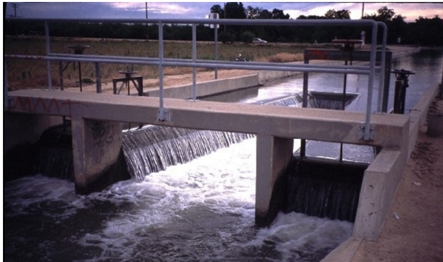
Figure 46. Somewhat similar LCW installed at Turlock ID
