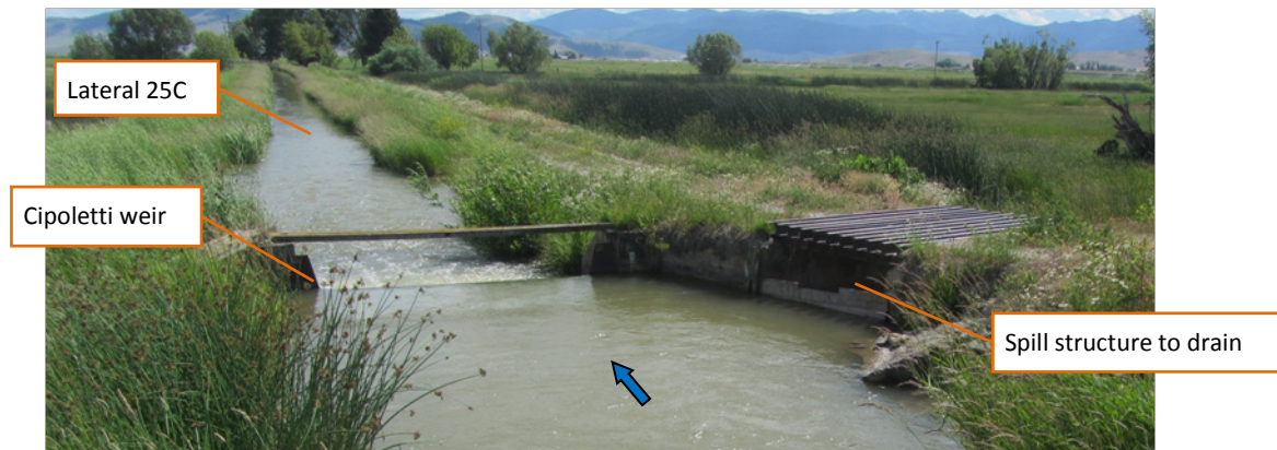
Figure 13. Existing Cipoletti weir and spill downstream of Lateral 25C head
