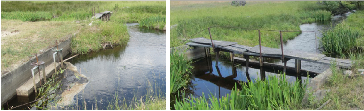
Figure 40. Existing 36F Canal headgates (left) and Dublin Gulch check structure (right)
