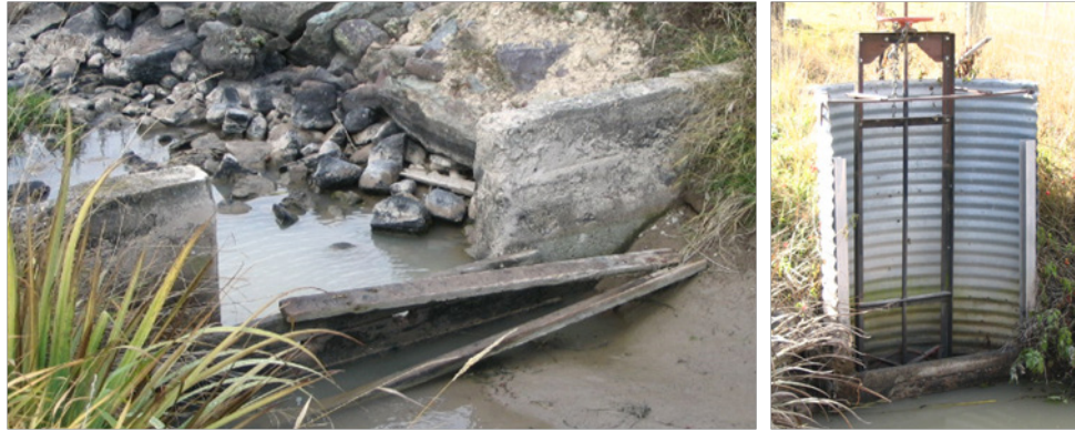
Figure 5. Existing Post B Canal check structure (left) and waste/spill structure gate (right) just west of Hall Road. Photos from HKM 2008 report.
