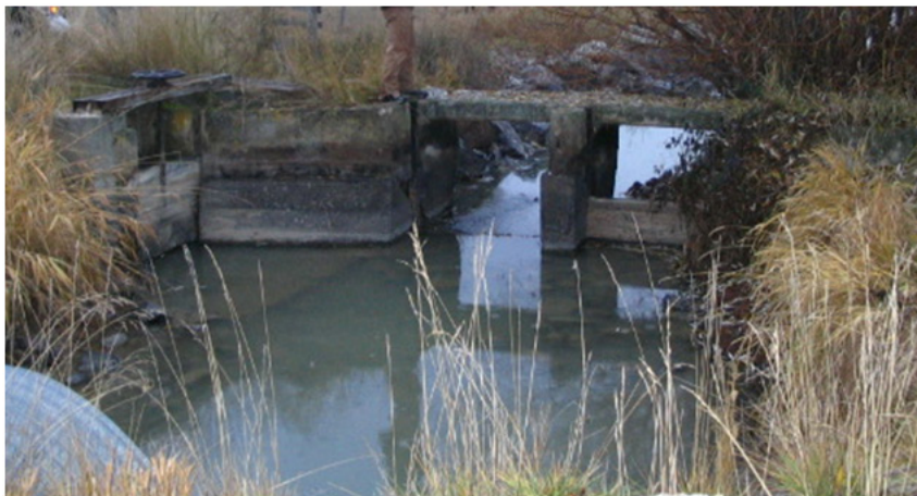
Figure 6. Existing check in Post C Canal, with the Lateral 22C headgate on the left-hand side
