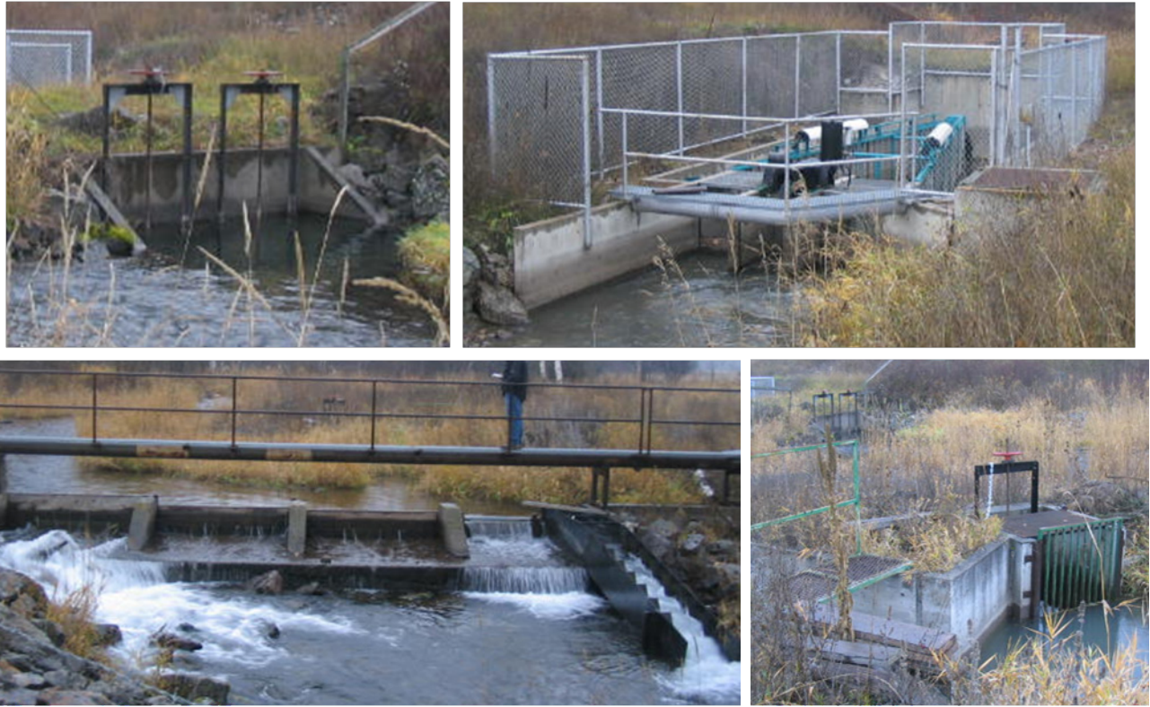
Figure 31. Post F Canal headgates (top left), Post F Canal fish screen (top right), Post Creek flashboard diversion (bottom left), Mission C Canal siphon entrance and waste (bottom right). Photos taken from HKM 2008 report.
