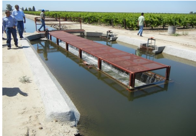
Figure 47. Somewhat similar LCW in Fresno ID, but lacking the side sluice gates and the tapered configuration of the LCW itself (although the banks are tapered). This illustrates a construction technique for tying the walls together for strength, and providing access for operators to clean off the weir crest.
