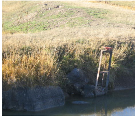
Figure 49. Existing manual waste gate on the Post F Canal. Photo from HKM 2008 report (CW-63).
