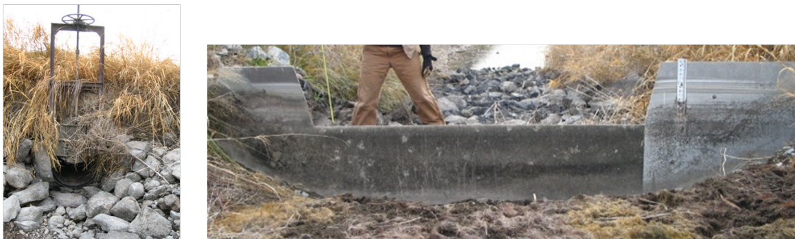
Figure 55. 24" Control gate into Post P Canal, and Cipoletti weir downstream of that gate. Photos provided from HKM 2008 report.
