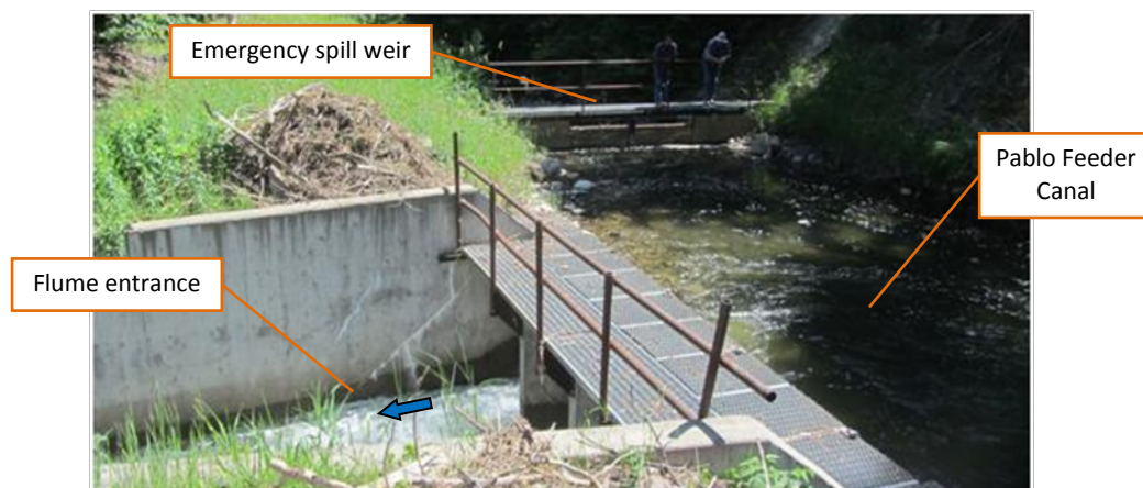
Figure 6. Pablo Feeder Canal flume entrance and emergency spill weir at Post Creek
