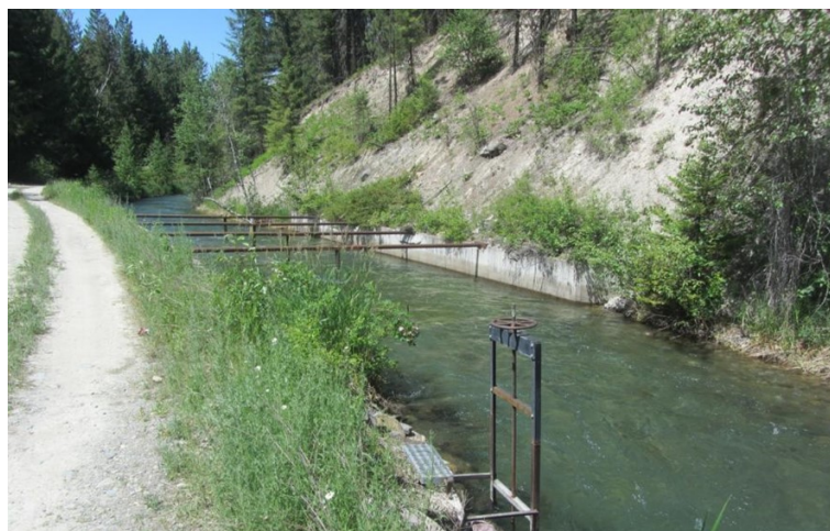
Figure 9. Pablo Feeder Canal and small gate to maintain instream flows; located downstream of the steel conveyance flume
