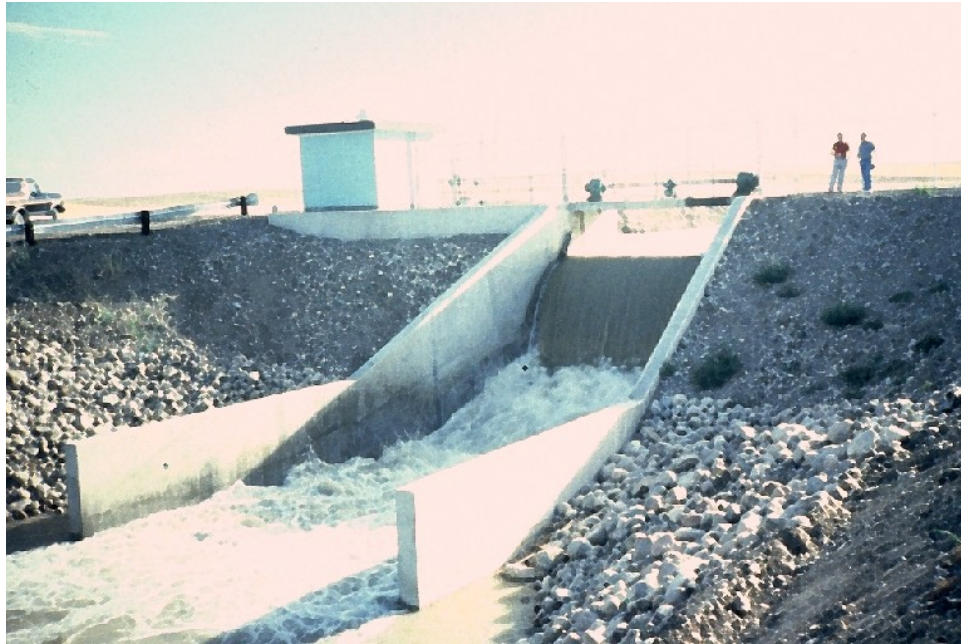
Figure 26. Example of an early automated overshoot gate near Lethbridge, Canada
