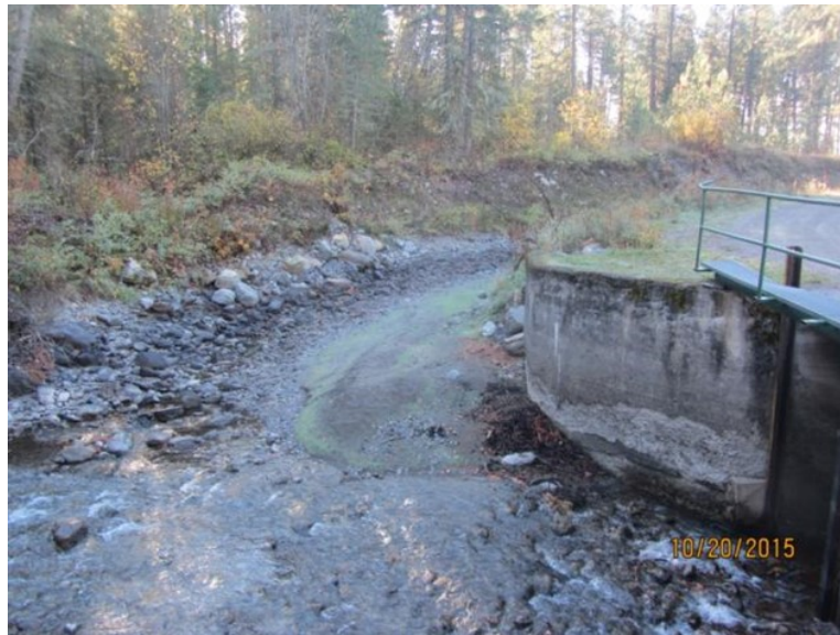
Figure 15. Confluence of South Crow Creek (entering from the left) and the Pablo Feeder Canal (entering from the top). Open flashboard structure plus canal gate on the right-hand side is a continuation of the South Crow Creek.
