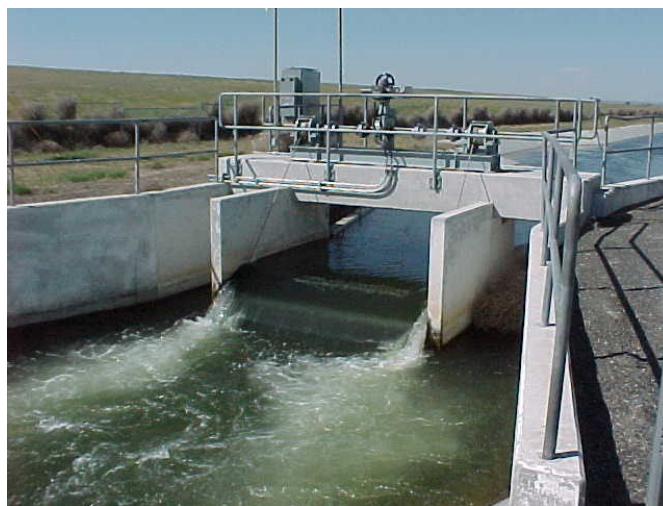
Figure 27. Hinged overshoot gate in a new structure, almost completely open. Umatilla, Oregon
