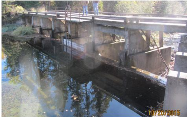
Figure 23. Seven bay check structure in North Crow Creek as the Pablo Feeder Canal passes through the pond
