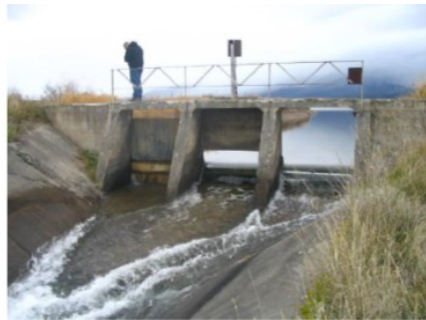
Figure 49. Structure at the head of the downstream section of the Kicking Horse Feeder Canal. View from downstream. Pond is seen upstream of the structure. Photo taken from HKM 2008 report.
