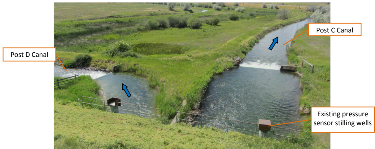
Figure 63. Existing Cipoletti weirs at the head of the Post C and D Canals at Ninepipe Reservoir
