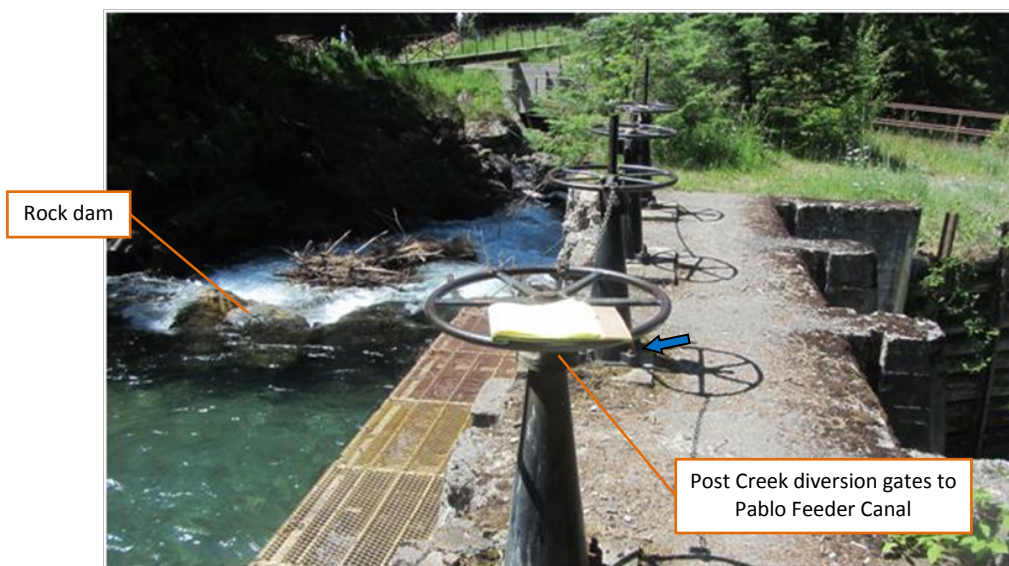
Figure 8. Rock dam in Post Creek, and diversion gates to supply the Pablo Feeder Canal
