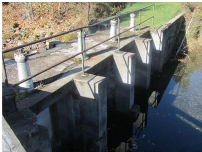
Figure 24. Existing manual flow control gates for the restart of the Pablo Feeder Canal at North Crow Creek
