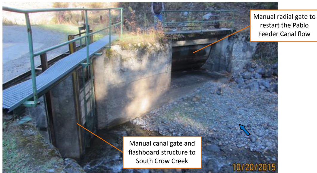
Figure 16. Existing structures in Pablo Feeder Canal at South Crow Creek
