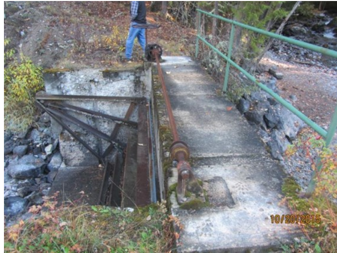
Figure 17. Radial gate to control flow into the Pablo Feeder Canal at South Crow Creek
