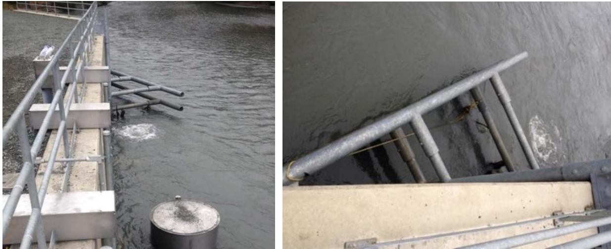
Figure 12. Views of horizontal trash deflector bars in a river
