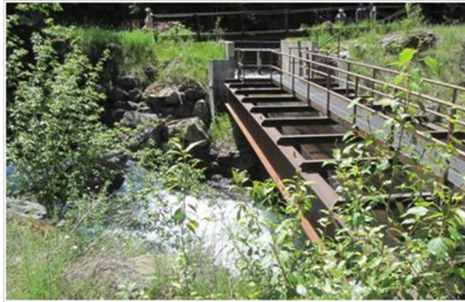
Figure 7. Pablo Feeder Canal steel flume over Post Creek
