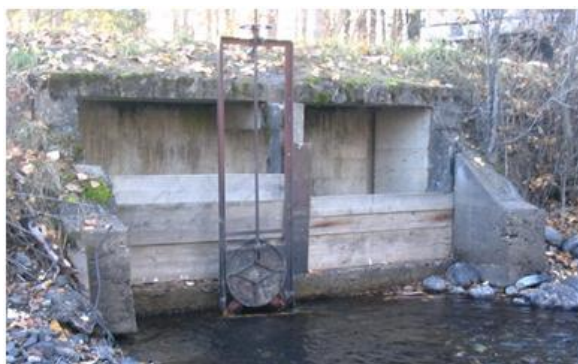
Figure 20. Existing spill structure in the Pablo Feeder Canal at Middle Crow Creek. Photo provided from HKM 2008 report.
