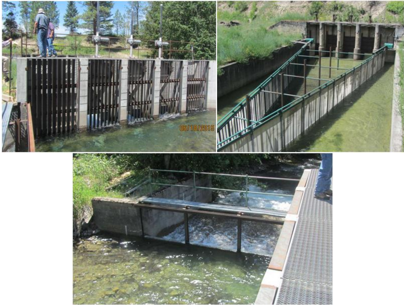
Figure 31. New canal headgates (top left), fish screen and old headgates (top right), Post Creek check structure (bottom) at the head of the Kicking Horse Feeder Canal
