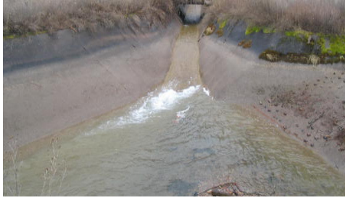
Figure 6. Existing concrete drop chute upstream of the headworks structures. Photo from HKM 2008 report (HW-5).
