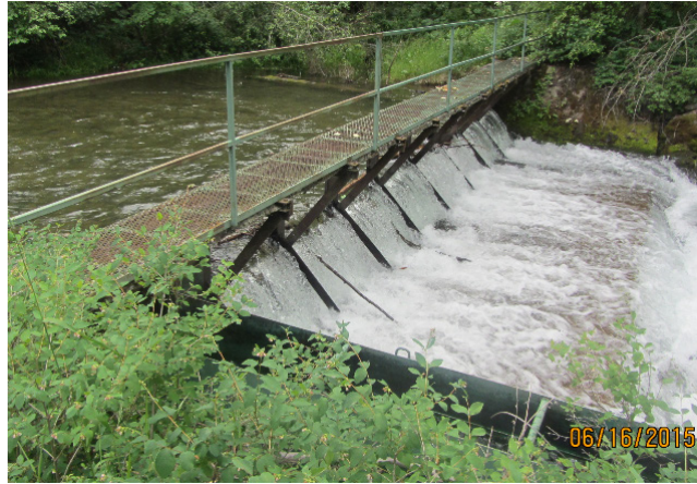
Figure 31. Existing diversion structure in Mission Creek for the Mission B Canal
