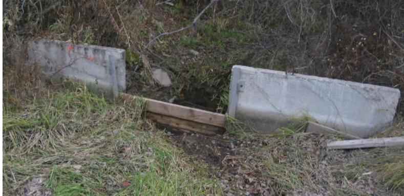
Figure 59. Existing 4' wide check/waste structure at the end of the Mission F Canal. Photo from HKM 2008 report (CW-74).
