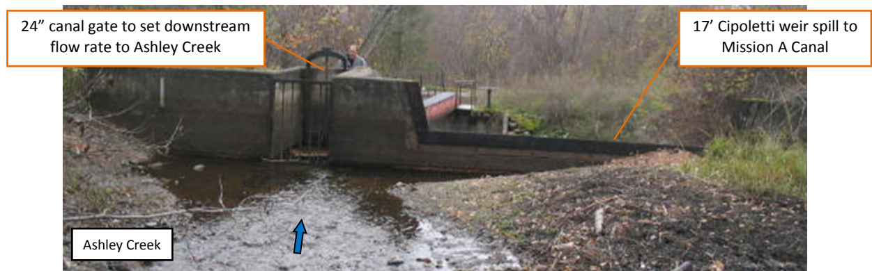
Figure 23. Upstream of Ashley Creek spill into the Mission A Canal. Photo from HKM 2008 report (CH-240).
