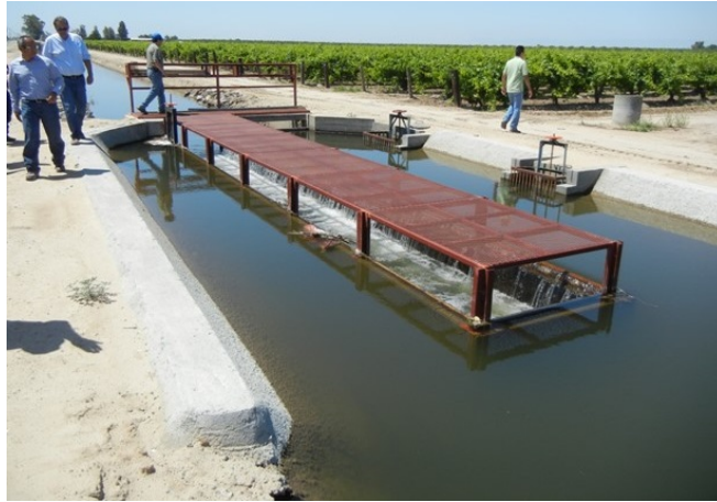
Figure 40. Somewhat similar LCW in Fresno ID, but lacking the side sluice gates and the tapered configuration of the LCW itself (although the banks are tapered). This illustrates a construction technique for tying the walls together for strength, and providing access for operators to clean off the weir crest.
