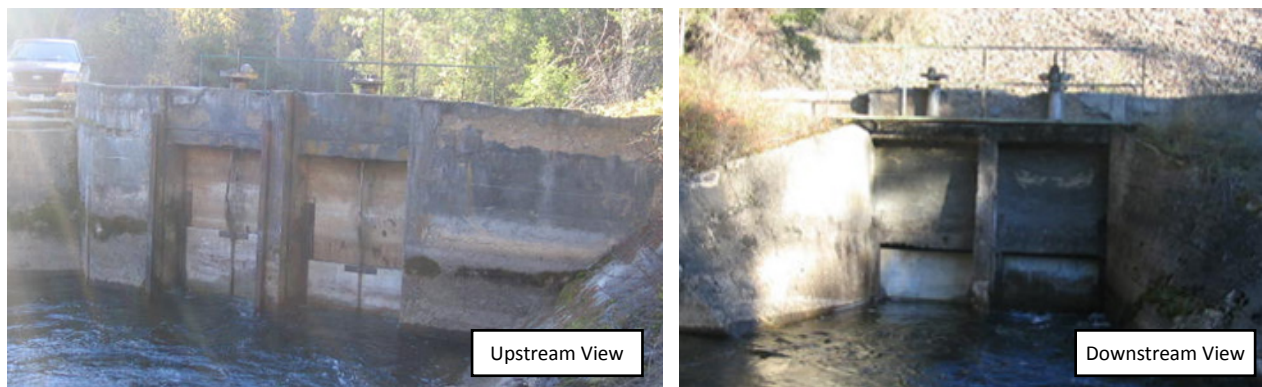
Figure 18. Two approximately 6' wide by 5' tall sluice gates to control the flow to the downstream portion of the Mission A Canal. Photo from HKM 2008 report (HW-9).
