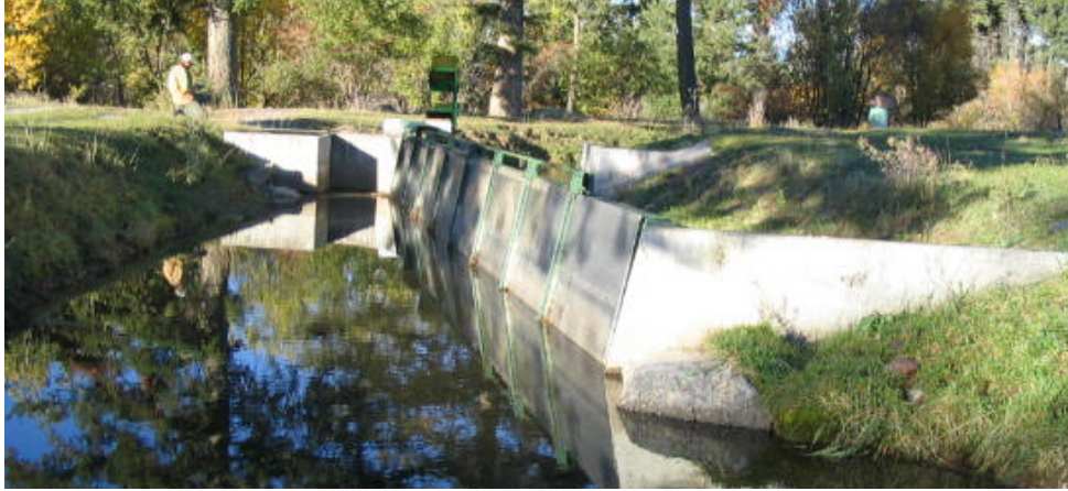
Figure 34. Existing fish screen in the Mission B Canal downstream from the canal head. Photo from HKM 2008 report (MSC-23).
