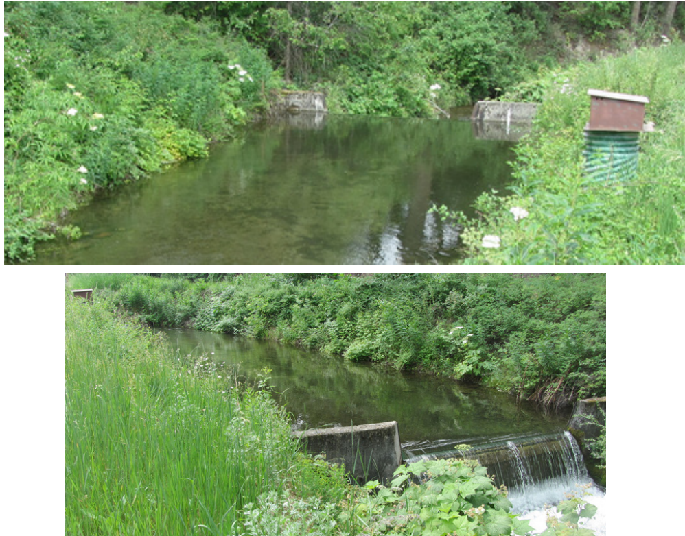
Figure 10. Existing 8' Cipoletti in the Mission F Canal for flow measurement
