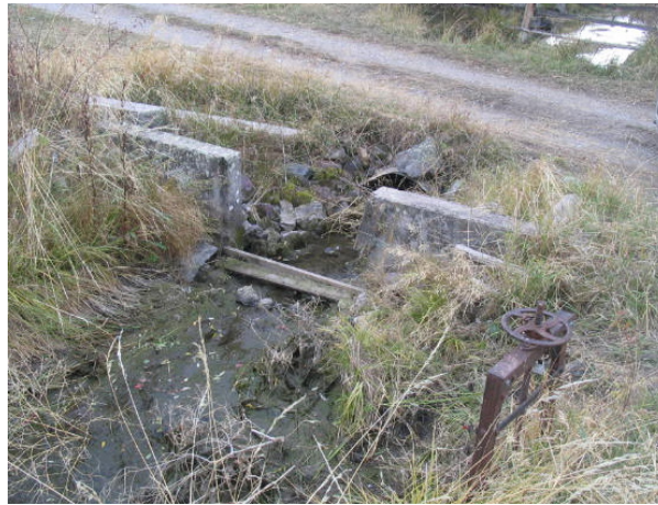
Figure 56. Example single bay flashboard check structure on the Mission F Canal. Photo from HKM 2008 report (CH-575).
