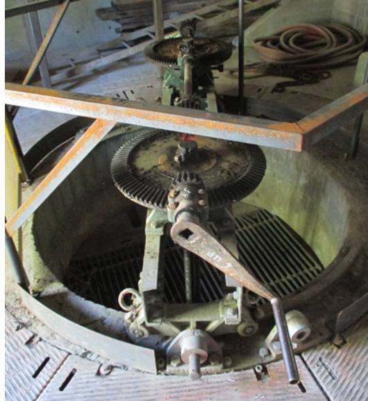
Figure 3. Existing Tabor Reservoir discharge cylinder gates
