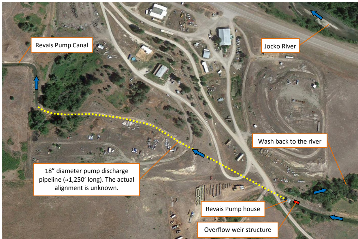
Figure 9. Aerial view of the existing Revais Pump System
