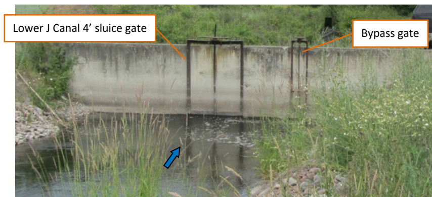
Figure 5. Lower J Canal headgate. It is unknown what the small gate is used for.
