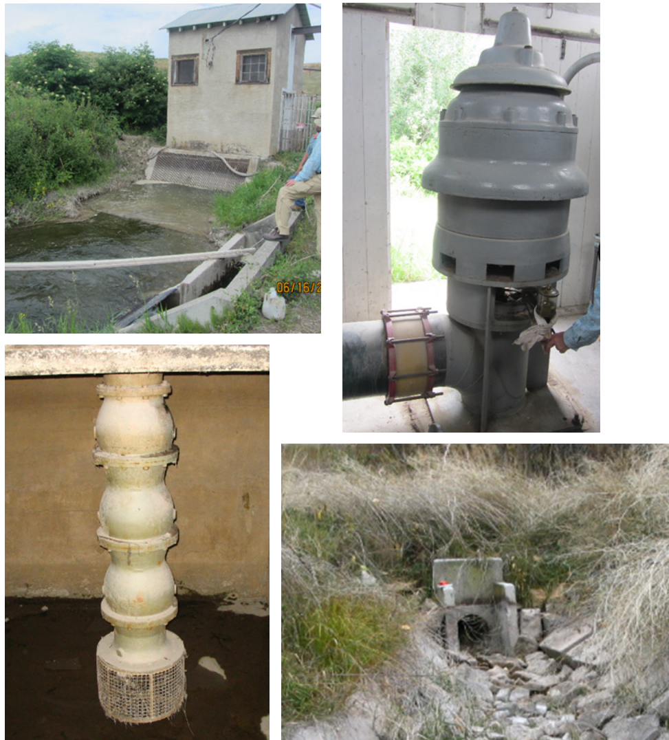
Figure 10. Revais Pump House (top left), Revais Pump (top right), three stage pump impellers (bottom left), and downstream of the pump discharge pipeline into the Revais Pump Canal (bottom right). Two bottom photos from HKM 2008 report.
