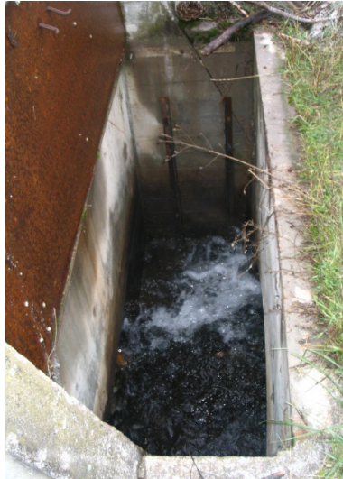
Figure 6. Open concrete box directly downstream of the Lower J Canal headgate wall. Photo from HKM 2008 report (HG-8).
