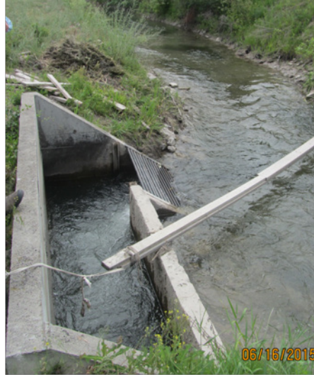
Figure 11. Existing Lower J Canal spill structure just upstream of Revais Pump
