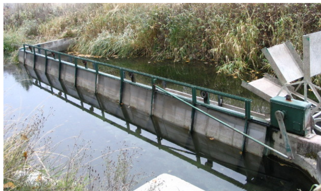
Figure 7. Existing fish screen in the Lower J Canal located approximately 100' downstream of the canal headgates. Photo from HKM 2008 report (MSC-17).
