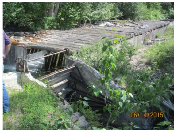
Figure 18. Existing Tabor Feeder Canal structure at Falls Creek
