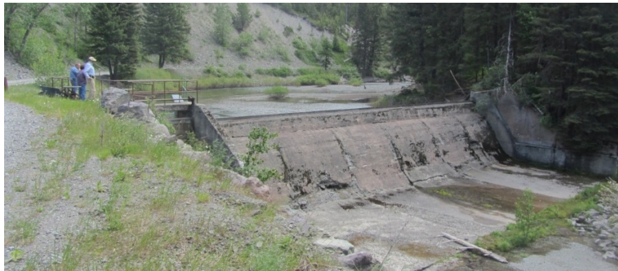
Figure 15. Tabor Feeder Canal diversion at North Fork Jocko River showing long weir dam and river bypass radial gate
