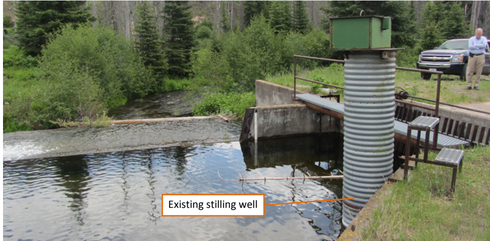
Figure 3. Existing Placid Canal diversion dam
