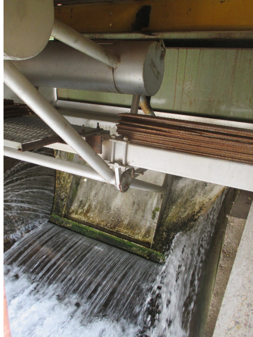
Figure 5. Existing AMIL gate downstream of the existing radial gate
