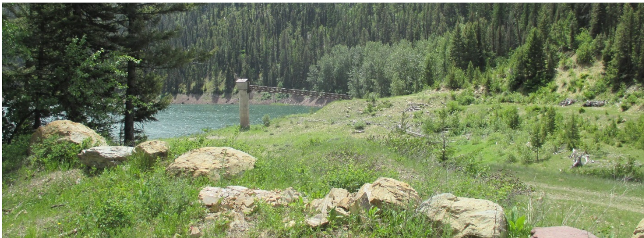
Figure 8. Lower Jocko Reservoir outlet gate and control building
