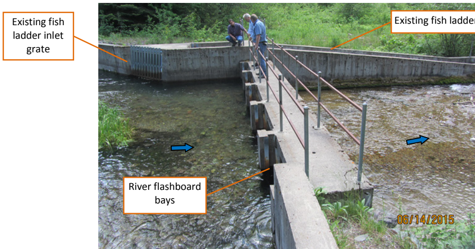
Figure 11. Existing Middle Fork Jocko River structures at the head of the Tabor Feeder Canal
