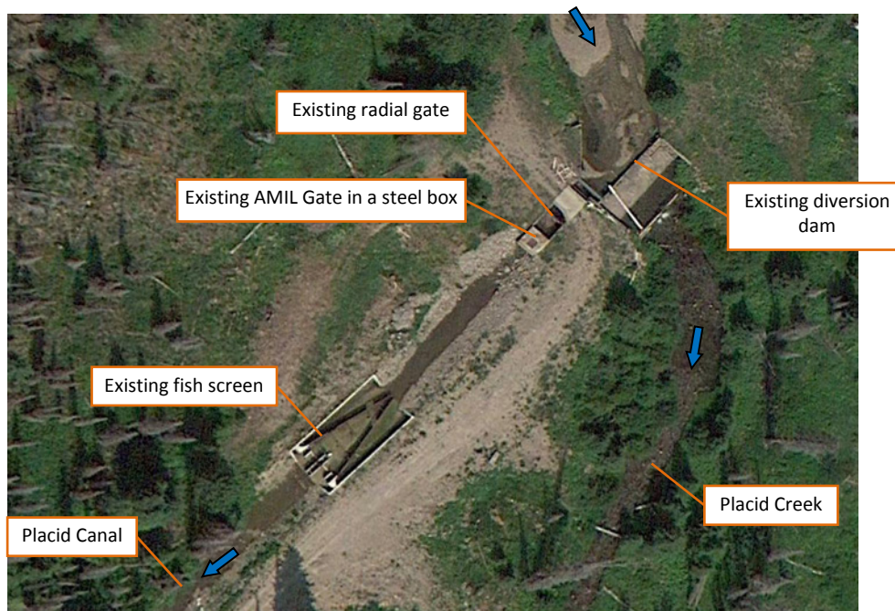
Figure 2. Aerial view of existing control at the head of the Placid Canal
