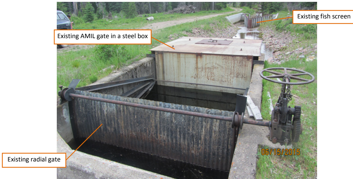
Figure 4. Existing Placid Canal headgate configuration
