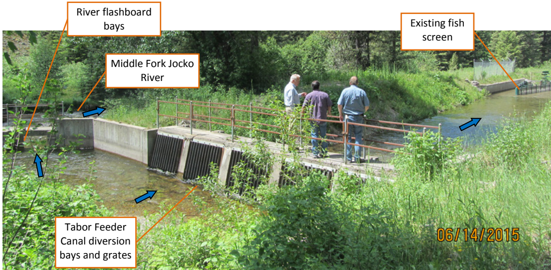
Figure 10. Existing infrastructure at the head of the Tabor Feeder Canal at Middle Fork Jocko River looking downstream
