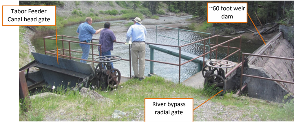
Figure 14. Existing infrastructure at the Tabor Feeder Canal diversion looking upstream at North Fork Jocko River
