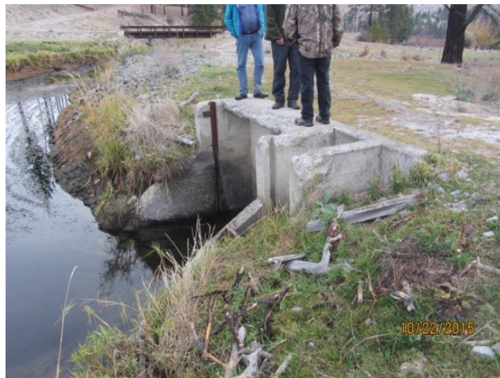
Figure 13. Inlet to the spill structure from the pond. The bridge in the background crosses the Camas A Canal, d/s of the tunnel exit. Mill Creek enters from the left-hand side of the photo.
