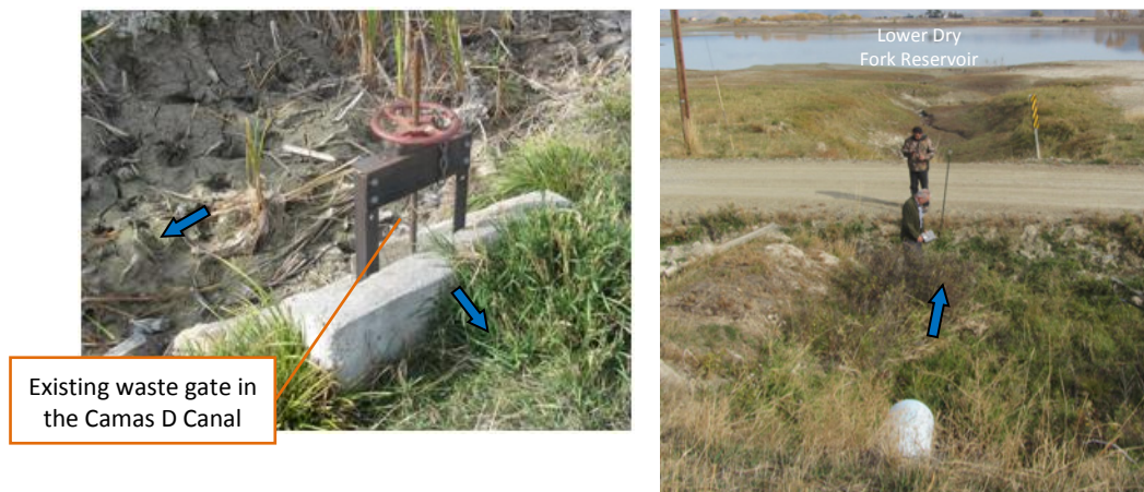
Figure 37. Existing Camas D Canal waste gate (left) and wash (right) to Lower Dry Fork Reservoir
