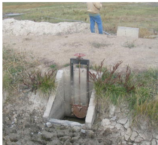
Figure 54. Manual waste gate that appears to service a nearby field. Photo from HKM 2008 report (CW-8).
