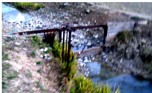
Figure 49. Existing check structure on the Camas C Canal located downstream of the proposed regulating reservoir site. Photo from HKM 2008 report (CH-26).
