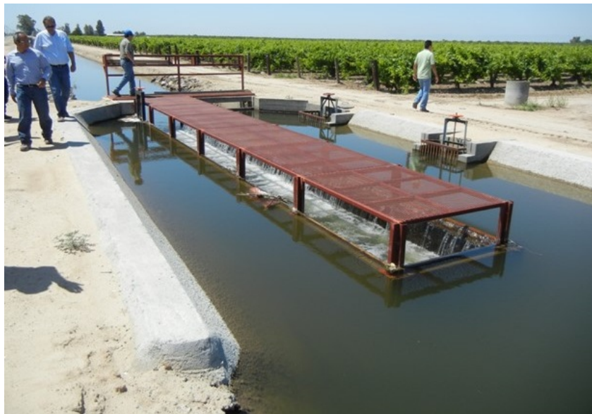
Figure 59. Somewhat similar LCW in Fresno ID, but lacking the side sluice gates and the tapered configuration of the LCW itself (although the banks are tapered). This illustrates a construction technique for tying the walls together for strength, and providing access for operators to clean off the weir crest.
