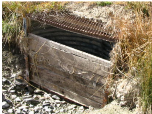
Figure 43. Existing waste check in the Camas B Canal immediately downstream of Kopp Rd. Photo from HKM 2008 report.
