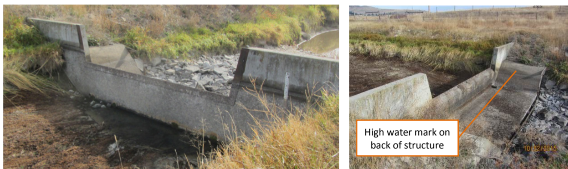
Figure 24. View of upstream side of 15' Cipoletti weir (left photo) and high water mark on downstream side of the weir (right photo) at head of Camas B Canal
