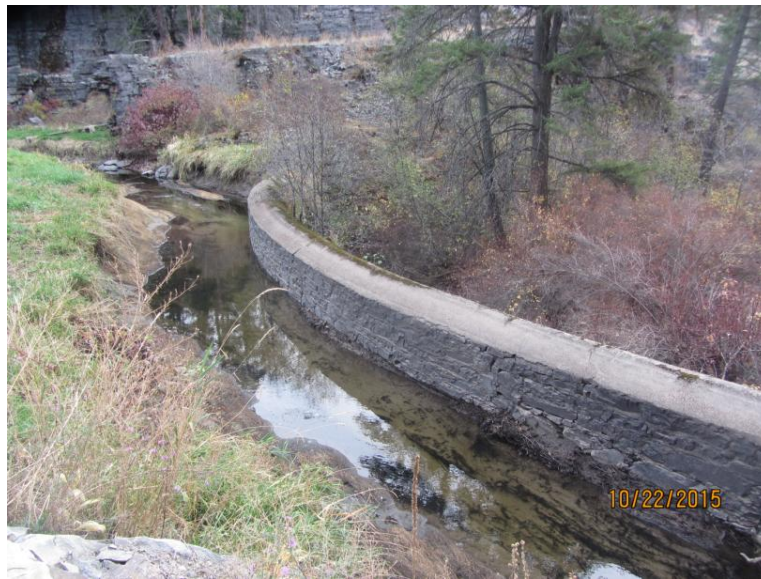
Figure 6. Upstream side of the masonry diversion dam
