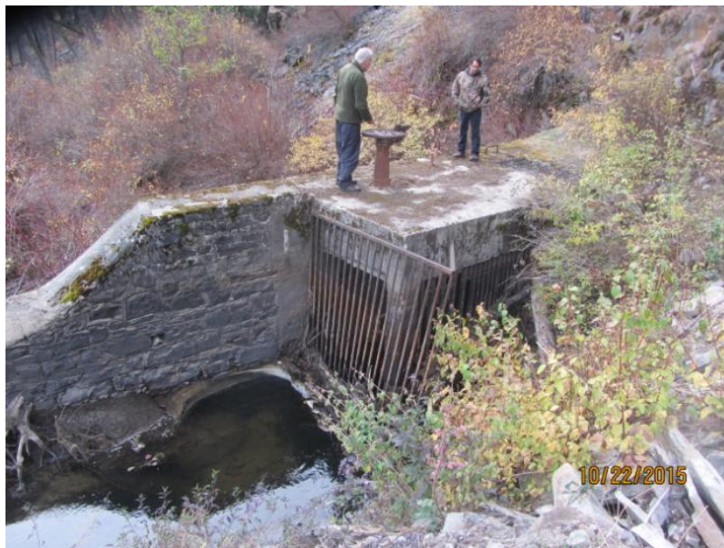
Figure 7. Inlet to the Camas A tunnel. Masonry dam is on the left. Sluice gate controls flow into downstream section of Lower Bitterroot Creek.
