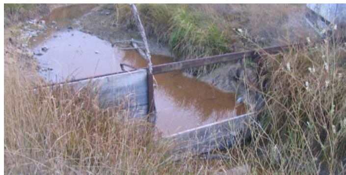
Figure 47. Existing check structure on the Camas C Canal located upstream of the proposed regulating reservoir site. Photo from HKM 2008 report (CH-25).
