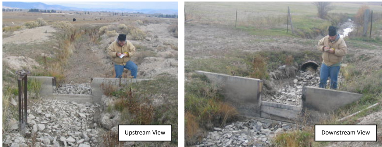
Figure 53. Last check structure on the Camas C Canal. Photos from HKM 2008 report (CD-4).
