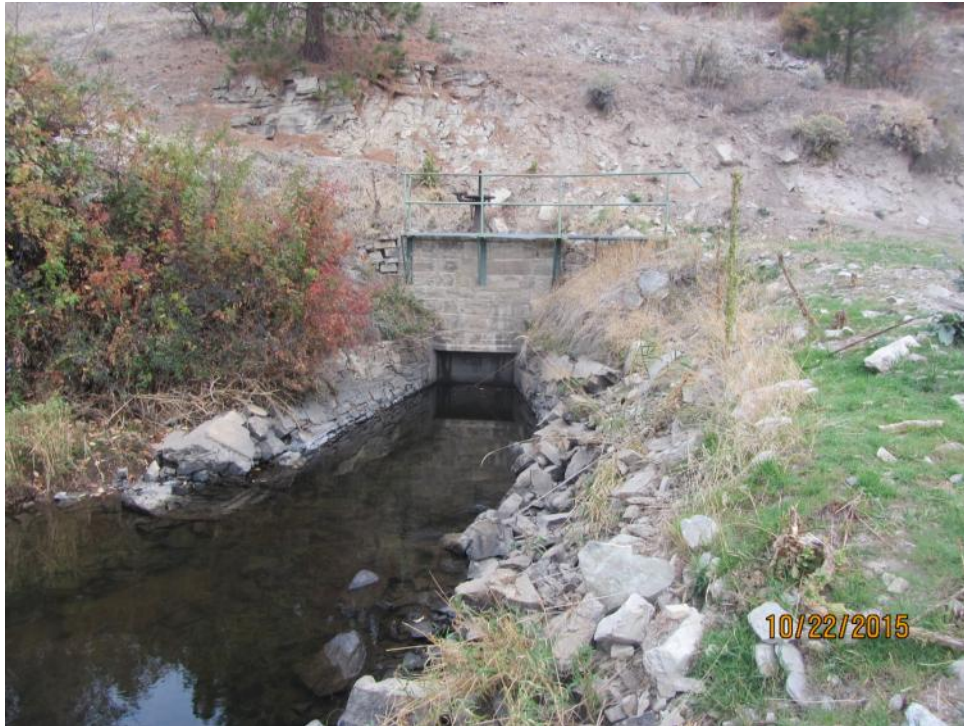
Figure 8. Manual sluice gate at the tunnel discharge
