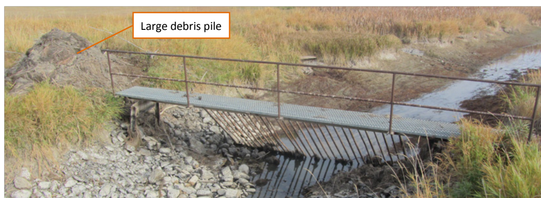
Figure 22. Existing trash rack upstream of Camas B and D Canal headgates
