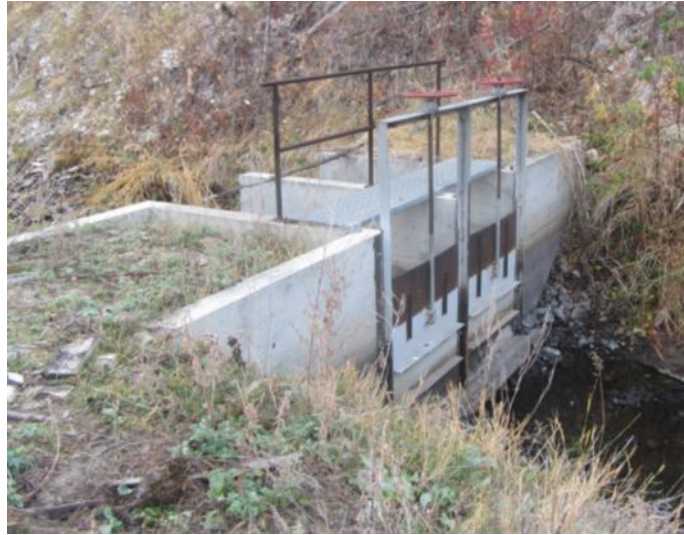
Figure 12. Existing Camas A Canal headgates near Mill Creek
