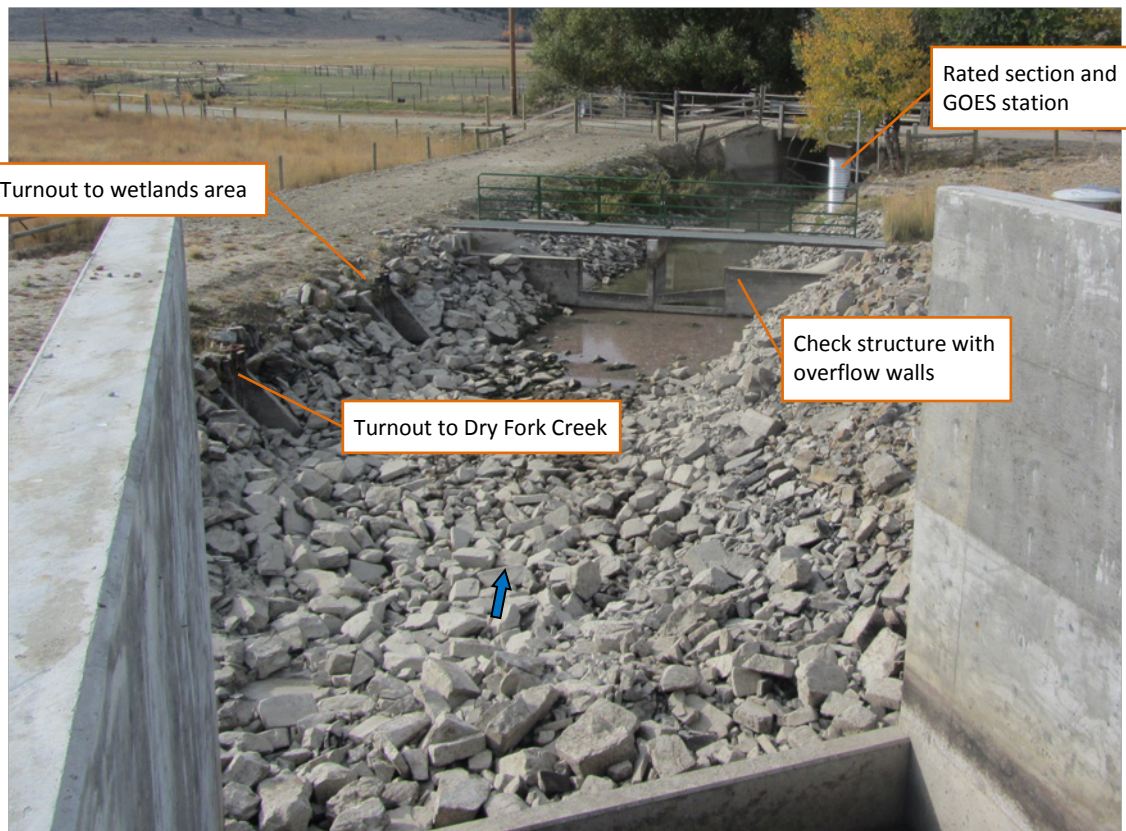
Figure 30. Existing control at the head of Camas C Canal at the outlet of Lower Dry Fork Reservoir
