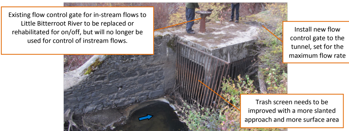
Figure 9. New flow control gate to the tunnel, at the Little Bitterroot River diversion
