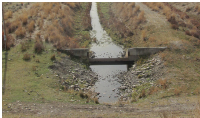
Figure 20. Existing approximately 15' rectangular weir downstream of Upper Dry Fork Reservoir outlet
