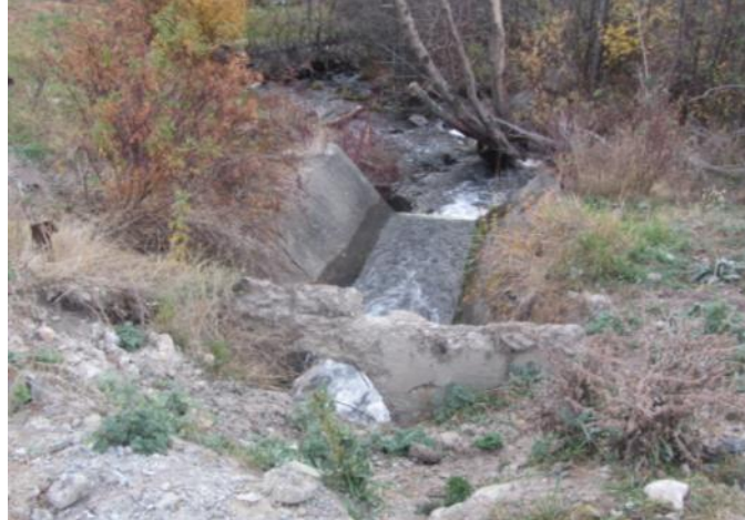
Figure 14. Downstream side of the spill structure from the pond
