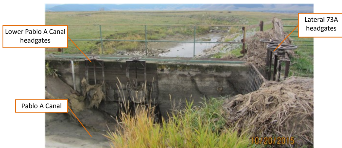
Figure 8. Existing Lower Pablo A Canal and Lateral 73A headgates
