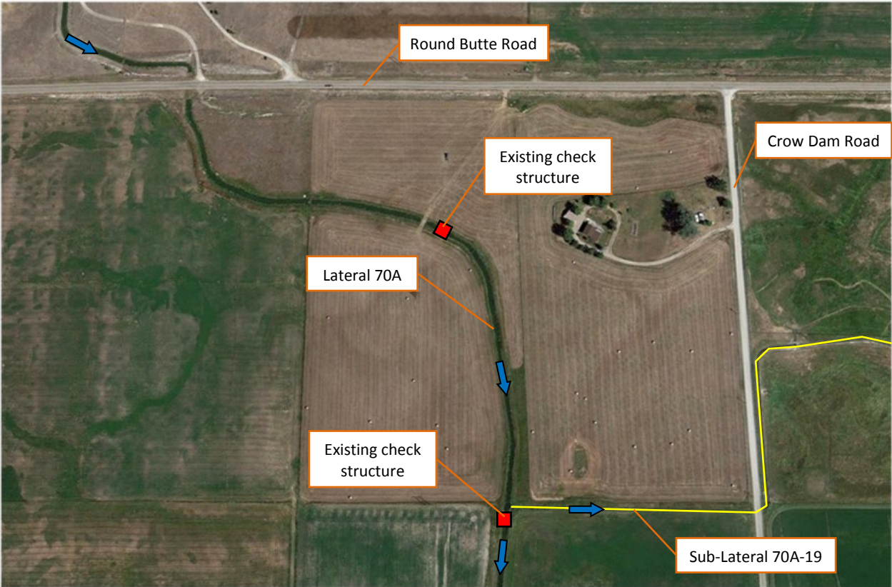
Figure 34. Existing conditions of Lateral 70A downstream of Round Butte Road
