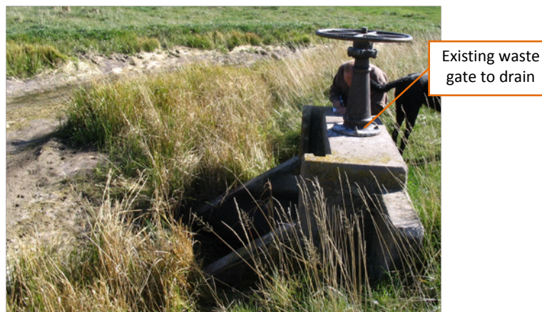
Figure 27. Existing waste gate to nearby drain. Photo from 2008 HKM report.
