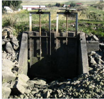
Figure 11. Existing Sub-Lateral 31A-1 headgates
