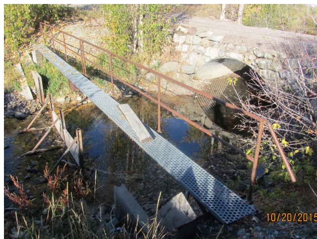
Figure 32. Existing check structure in the Pablo Feeder Canal located downstream of Dubay Road
