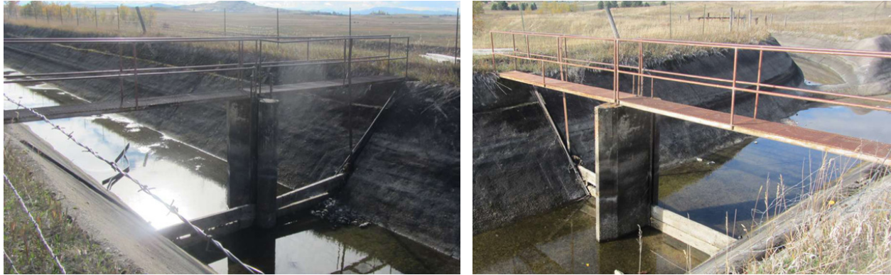
Figure 17. Upstream (left) and downstream (right) views of the existing check structure located downstream of the Pablo Drop
