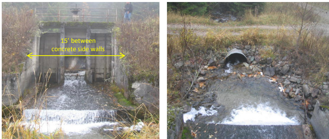
Figure 42. Downstream of the Mud Creek Diversion headgate on the Pablo Feeder Canal. Photos from HKM 2008 report (HW-25).
