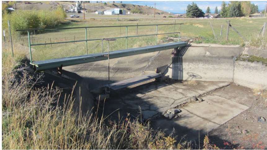
Figure 27. Existing manual check gate at head of the chute drop in the Pablo Feeder Canal upstream of Highway 93
