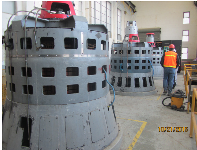
Figure 4. The three individual Flathead River Pump motors
