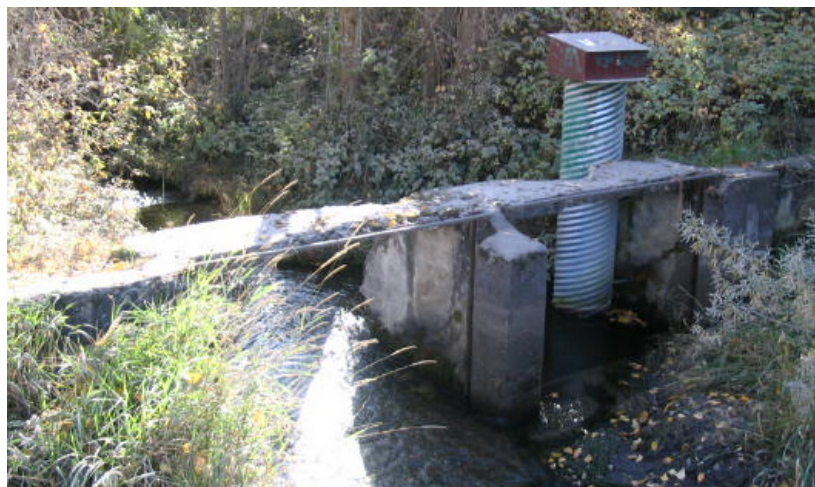
Figure 45. Existing check structure in Mud Creek just downstream of the Ronan B Canal headgates. Photo from HKM 2008 report (CH-466).
