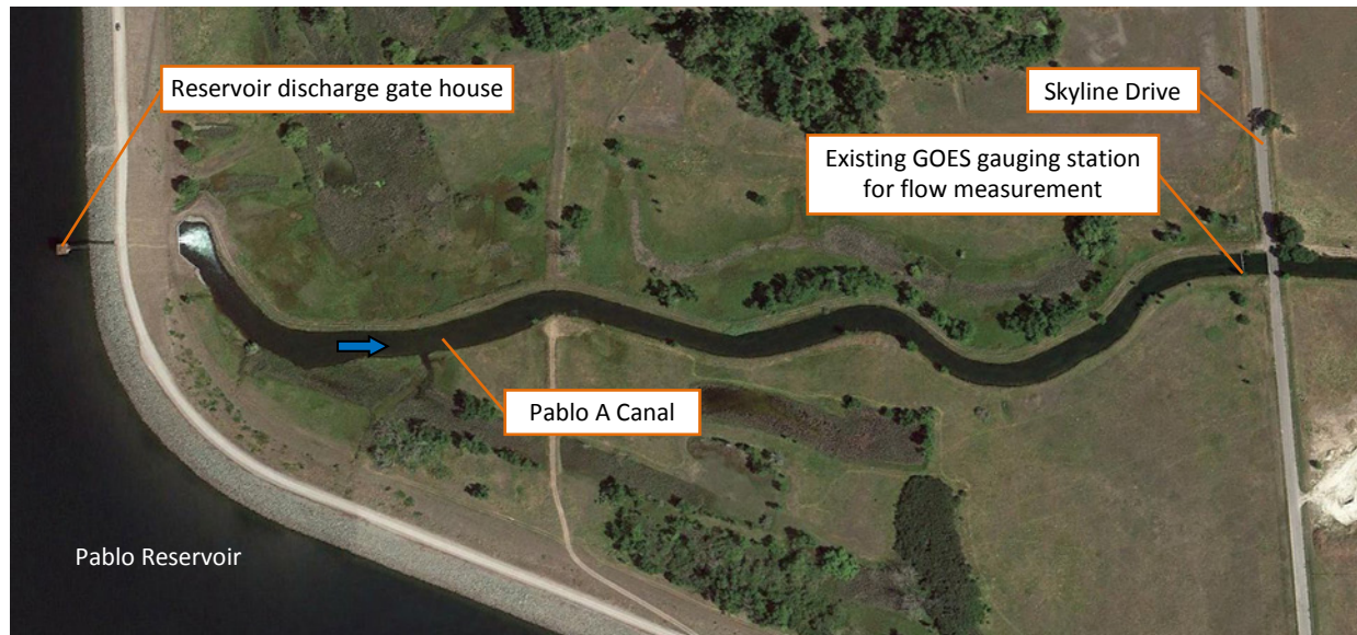
Figure 37. Existing conditions at the discharge of the Pablo Reservoir into the Pablo A Canal
