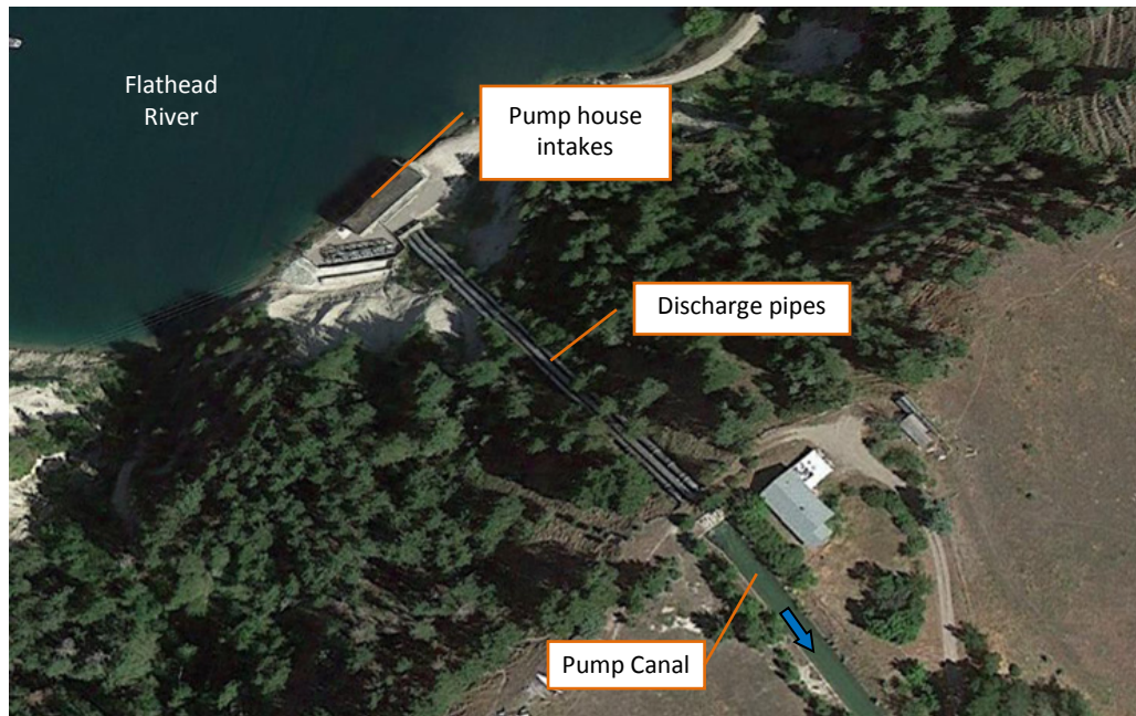
Figure 2. Aerial view of the Flathead River Pump House and its discharge into the Pump Canal
