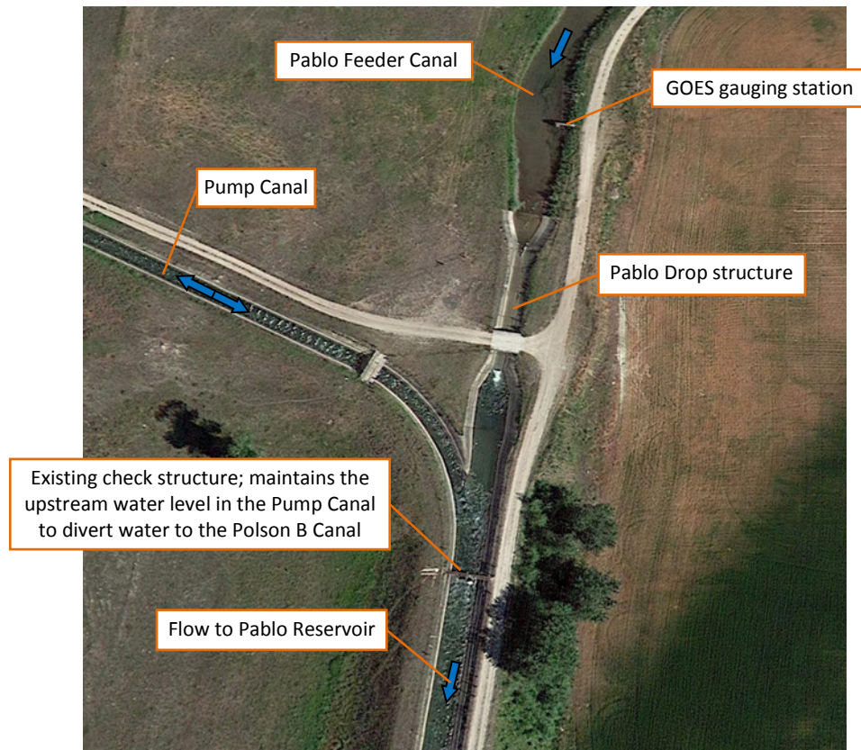
Figure 14. Existing conditions at the Pablo Drop
