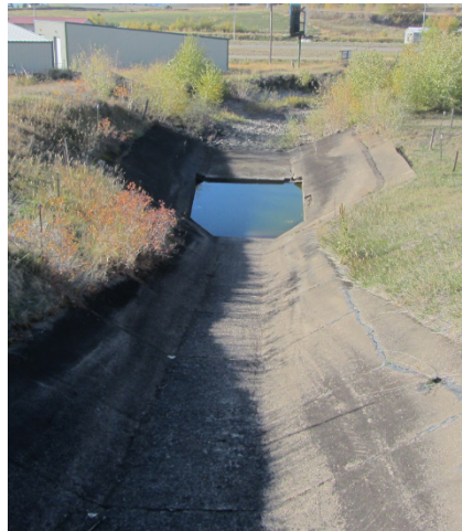
Figure 28. Chute drop on the Pablo Feeder Canal upstream of Highway 93
