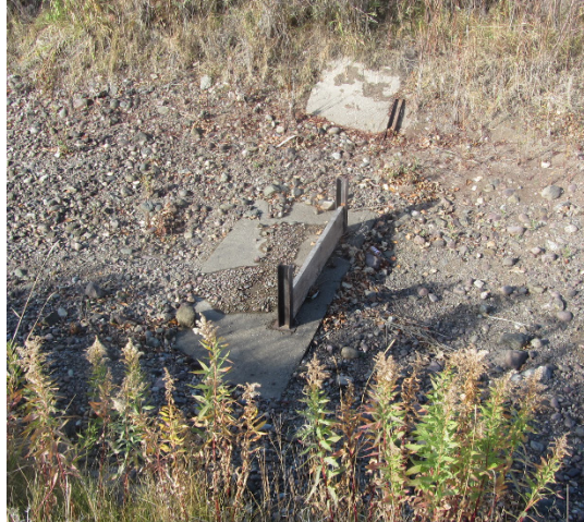
Figure 22. Small check in the Pablo Feeder Canal upstream of Caffrey Rd.
