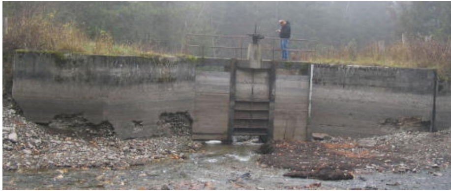
Figure 41. Mud Creek headgate on the Pablo Feeder Canal. Photo from HKM 2008 report (HW-25).
