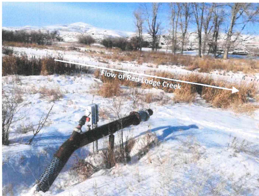
Figure 1: Intake of buried pipeline at pump site in the NENESE of Section 5, T5S R20E, December 16, 2022.
