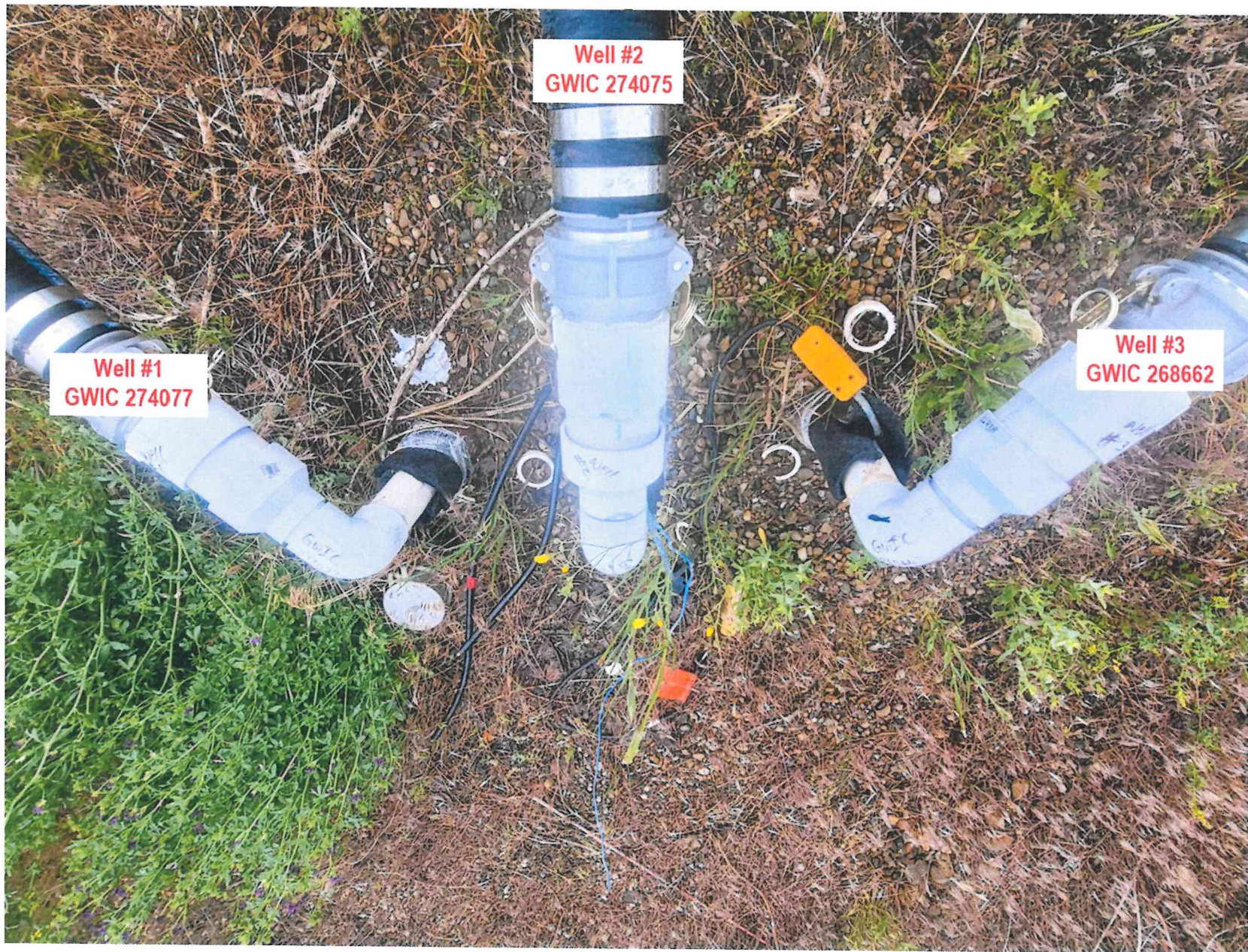
This photo shows all 3 wells exposed at surface at the manifold area. From here each well is connected to the manifold by a piece of 4 inch pipe.
