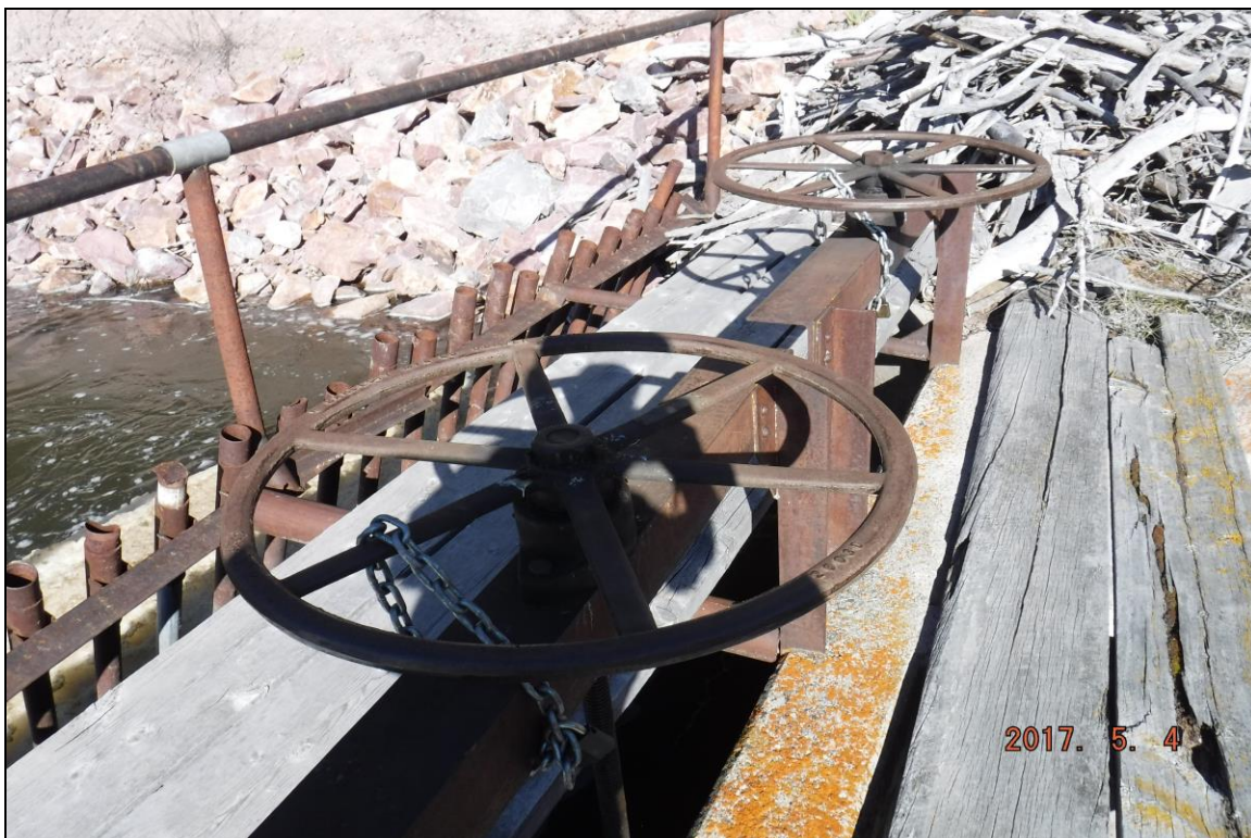
Looking W at gate wheels of the existing diversion structure in the Allendale Canal.
