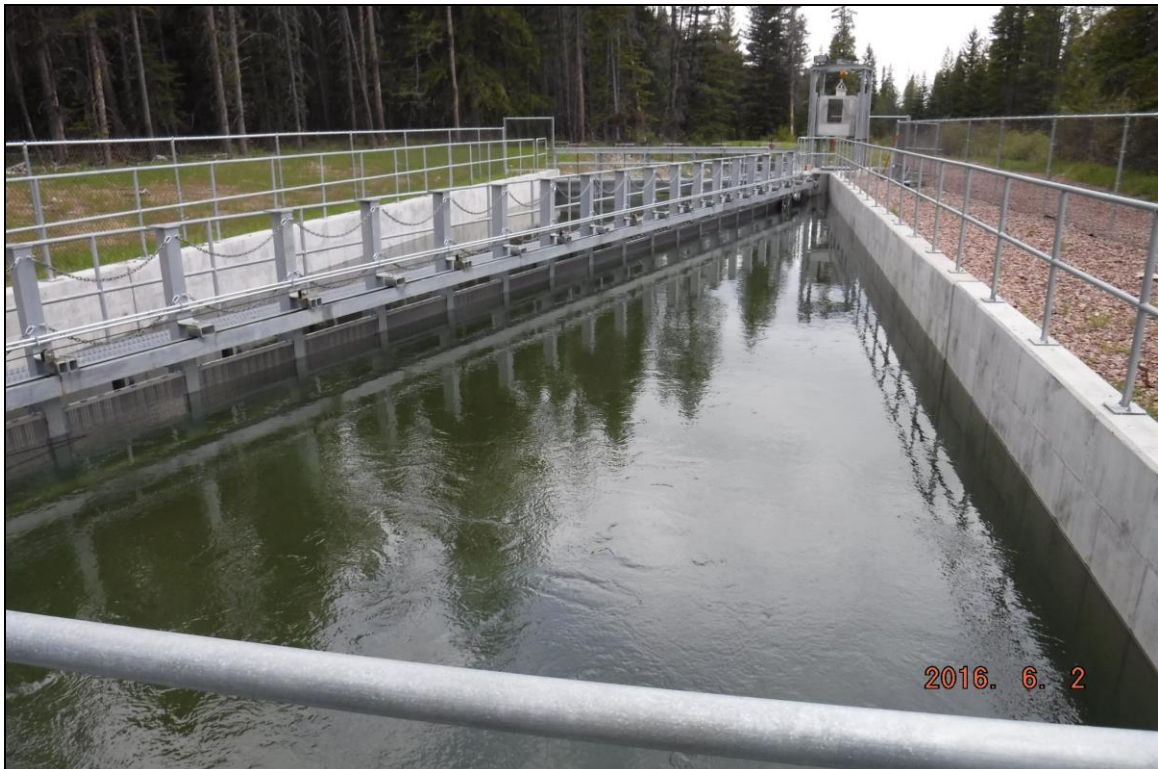
Example of the type of fish screen proposed for the Allendale Canal.
