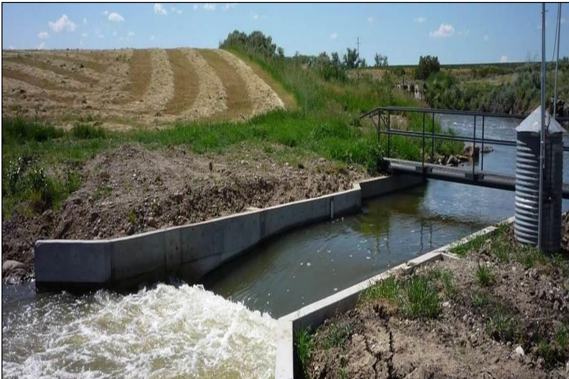
Example of weir/flume type structure to be installed in the Allendale Canal.
