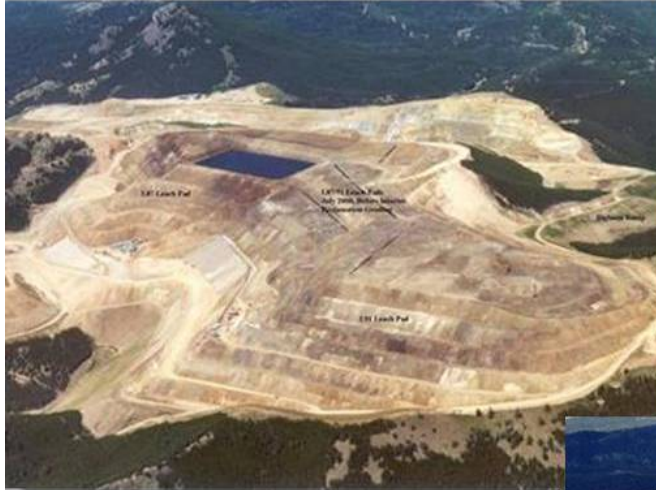
July 2000 - L87/91 Valley-Fill Leach Pads. Contains 112 million tons of spent ore, over 150 million gallons of residual cyanide solution and covers over 200 acres.
