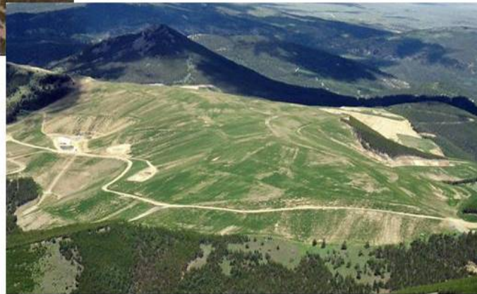
June 2006 - L87/91 Leach Pad After regrading, topsoil placement and seeding. Third year vegetation.
