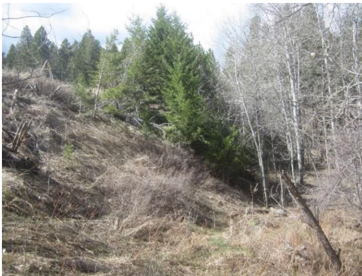
Trees on downstream embankment at critical section.
