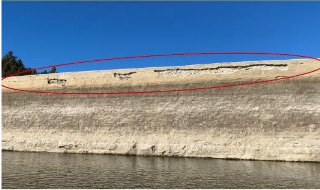
View of general concrete deterioration along upper face of Basin Creek Dam.
