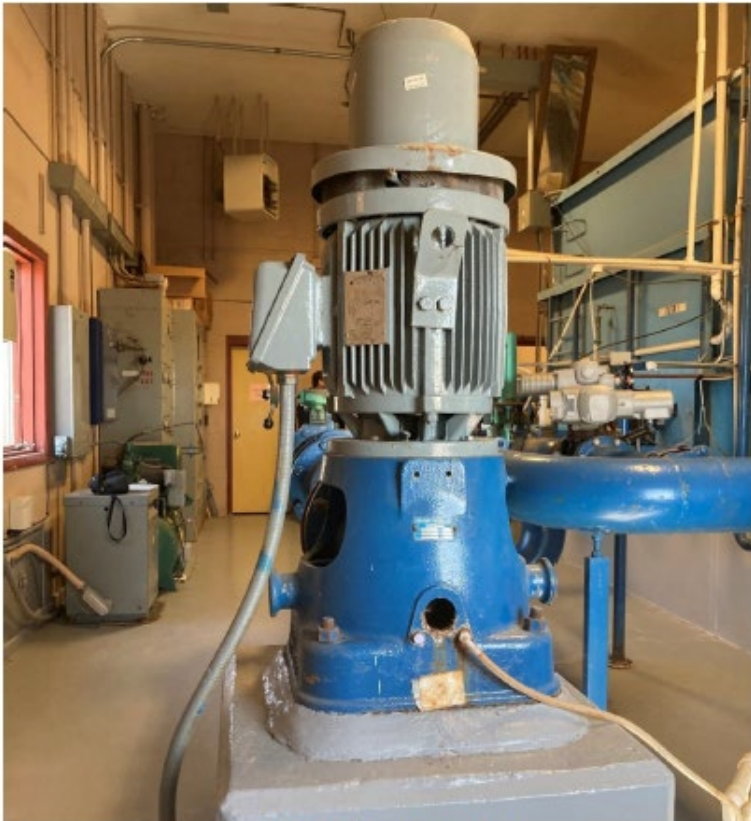
Filter backwash pump
