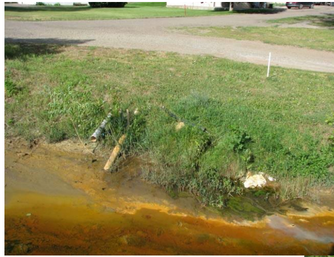
Mine drainage pipes in the District to more groundwater away from homes
