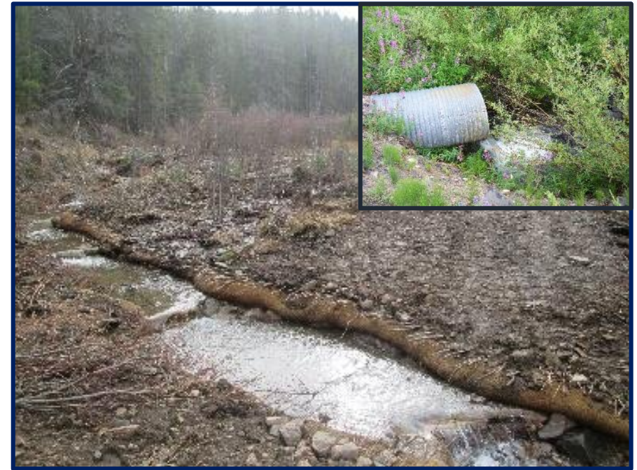
Step-pool feature at top of project after culvert removal (inset image of culvert from 2014)
