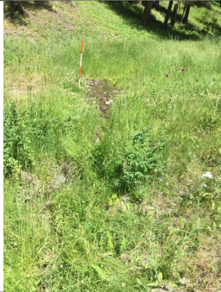
View of existing ford crossing at Project Site #1 looking upstream (date: July 2022).
