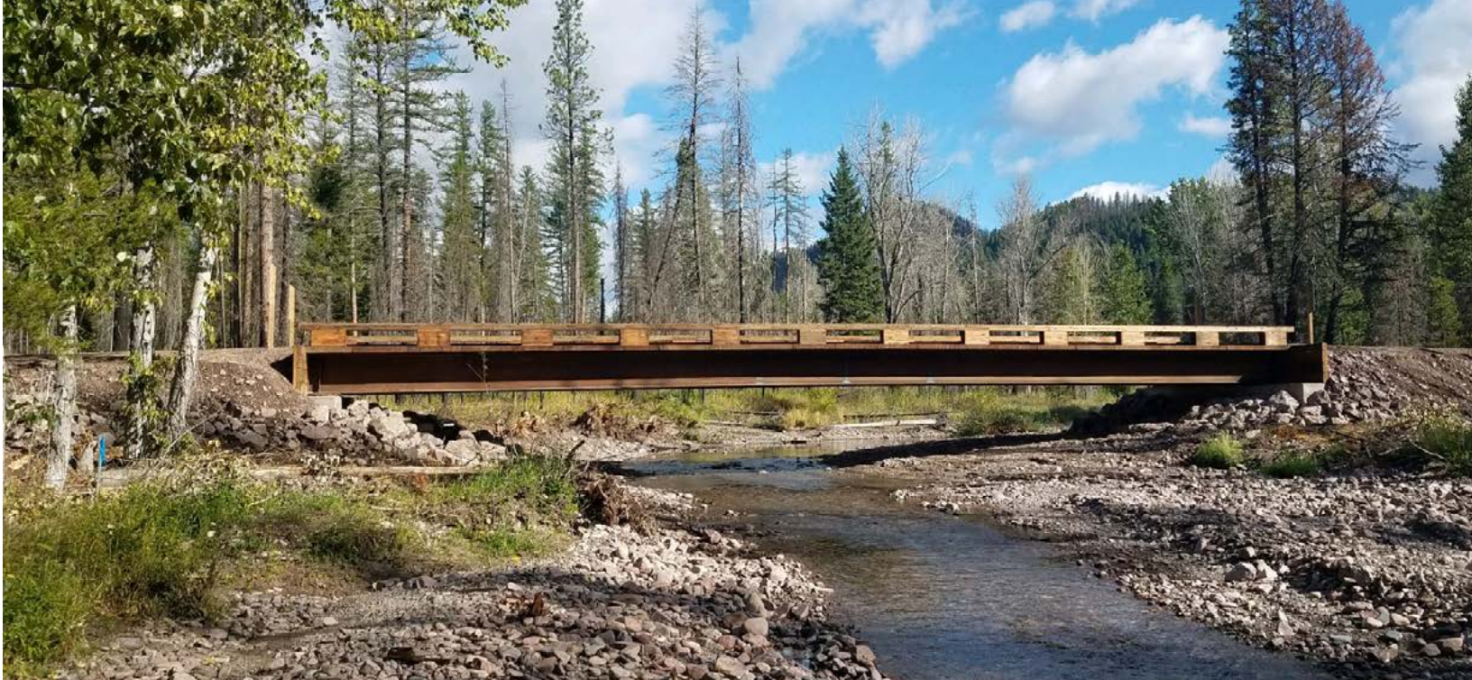
Installation of Aquatic Organism Passage structures increase ecological connectivity and improve watershed condition, while also protecting infrastructure to withstand flooding, run-off, or future debris flows. / Photo by USDA FS
