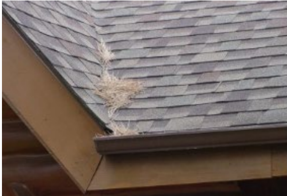
Figure 6.3. Examples of an uncovered gutter at risk of ignition (left) due to flammable tree debris, and a less-ignitable gutter (right) with a noncombustible gutter guard.
