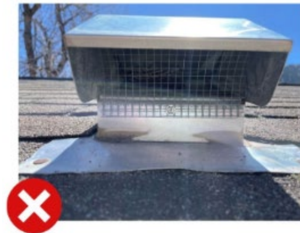
Figure 6.4. Examples of a bad vent (left) with 1/4-inch mesh that is ineffective at preventing ember incursion, and a good vent (right) that has 1/8-inch mesh to help prevent embers from entering the home.
