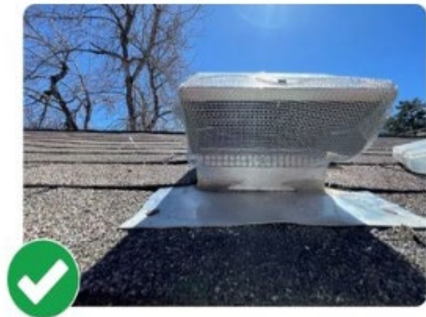
Figure 6.4. Examples of a bad vent (left) with 1/4-inch mesh that is ineffective at preventing ember incursion, and a good vent (right) that has 1/8-inch mesh to help prevent embers from entering the home.
