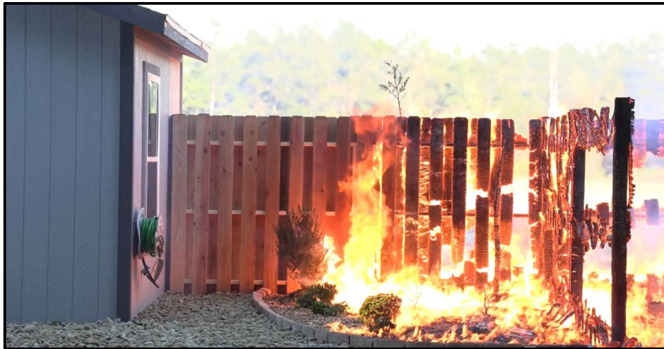
Figure 6.6. Example of combustible back-to-back fencing ignited by the fuels between and around them.
