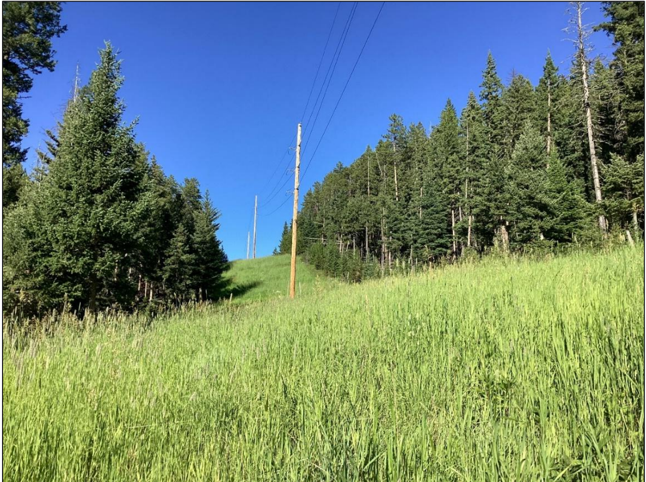
Figure 36: Example of a Non-Shaded Fuel Break
