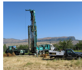
Main Harbor Well Drilling
