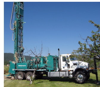
Main Harbor Well Drilling, Mike Lein
