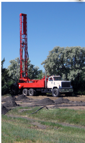
Iba Drilling, geothermal wells, Havre
