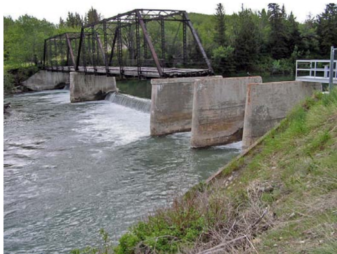
St. Mary diversion dam and bridge
