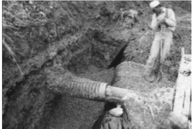
Installing diaphragm filter around slip-lined pipe on Dogget Dam
