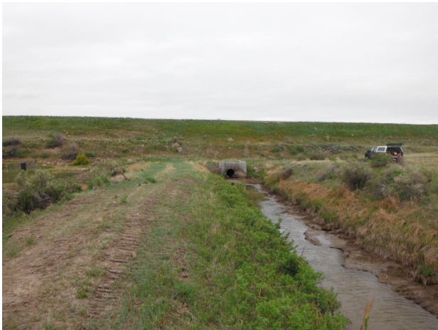
Outlet and downstream face of dam
