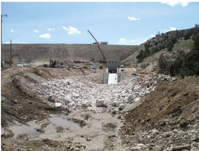
Outlet works under construction
