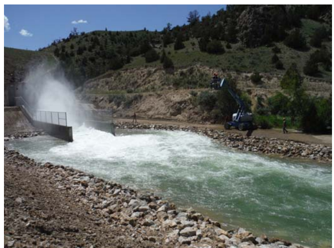
Outlet Works Operational Test
