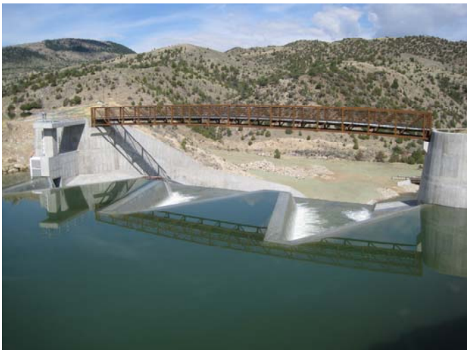
Labyrinth weir spillway and footbridge
