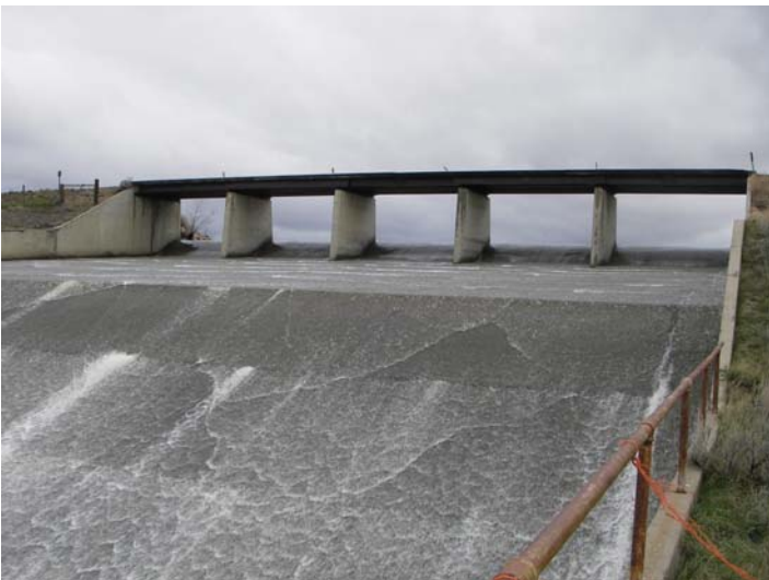
Spillway and county road bridge
