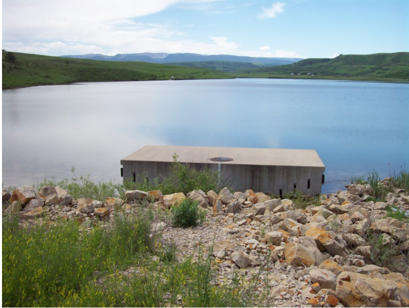
PHOTO 2-1. EAST FORK DAM, LEWISTOWN, MONTANA.
