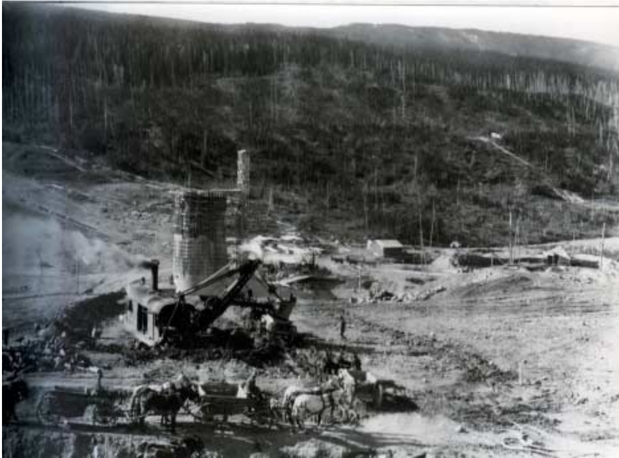
Construction of Outlet Tower at Sherburne Dam. Circa 1915 - Courtesy of USBR
