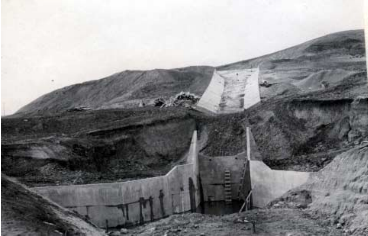
Construction of chute and pool at Drop #4. Courtesy of USBR
