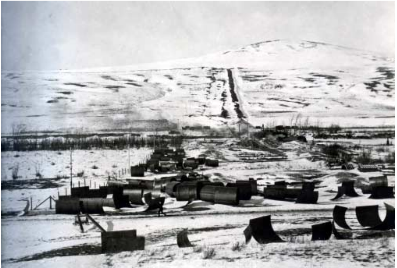
Steel for St. Mary River siphons. Circa 1912-1915 - Courtesy of USBR
