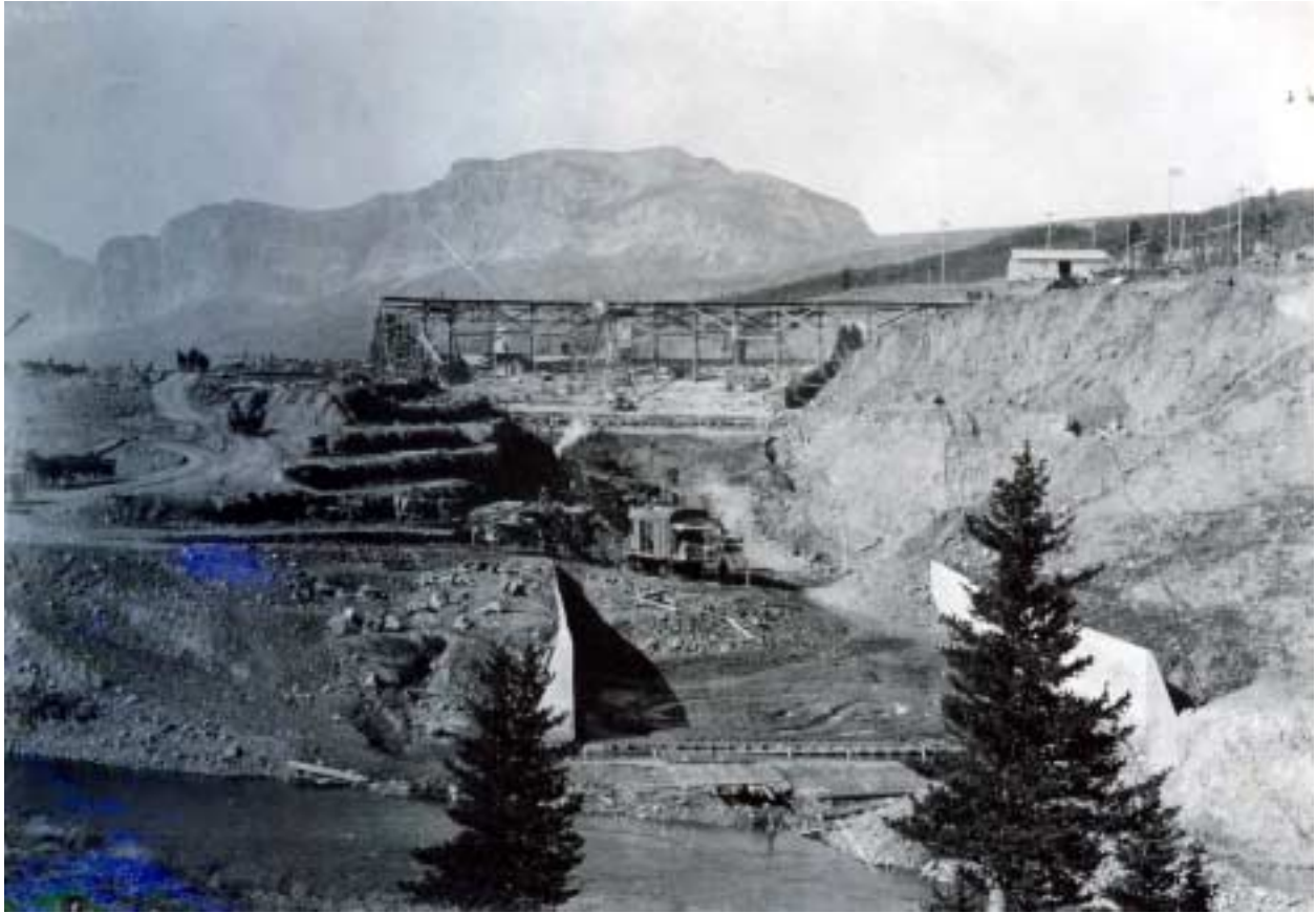
Construction of spillway channel on Sherburne Dam. Circa 1915 - Courtesy of USBR
