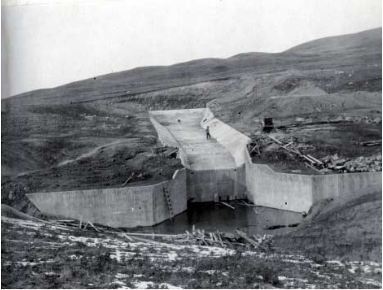
Completion of Drop #2. Courtesy of USBR
