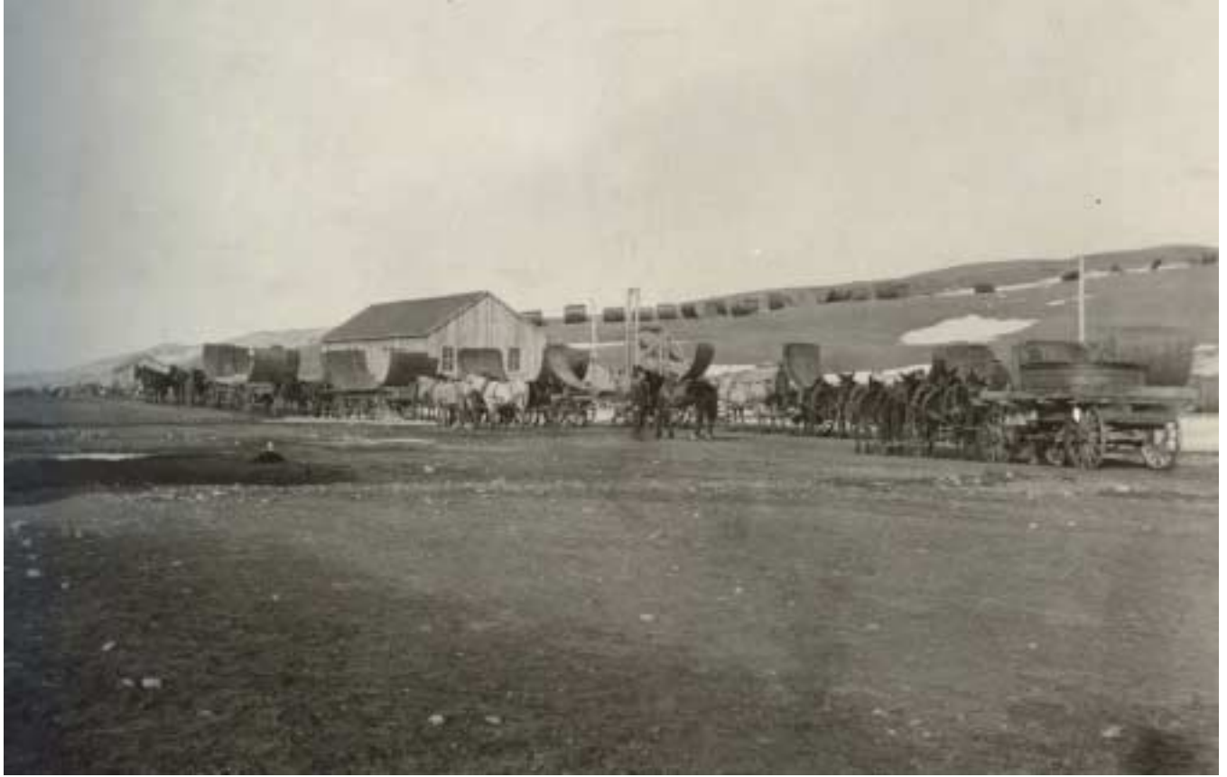
Steel for St. Mary River siphons were brought to the site by mule teams. Circa 1912-1915 - Courtesy of USBR
