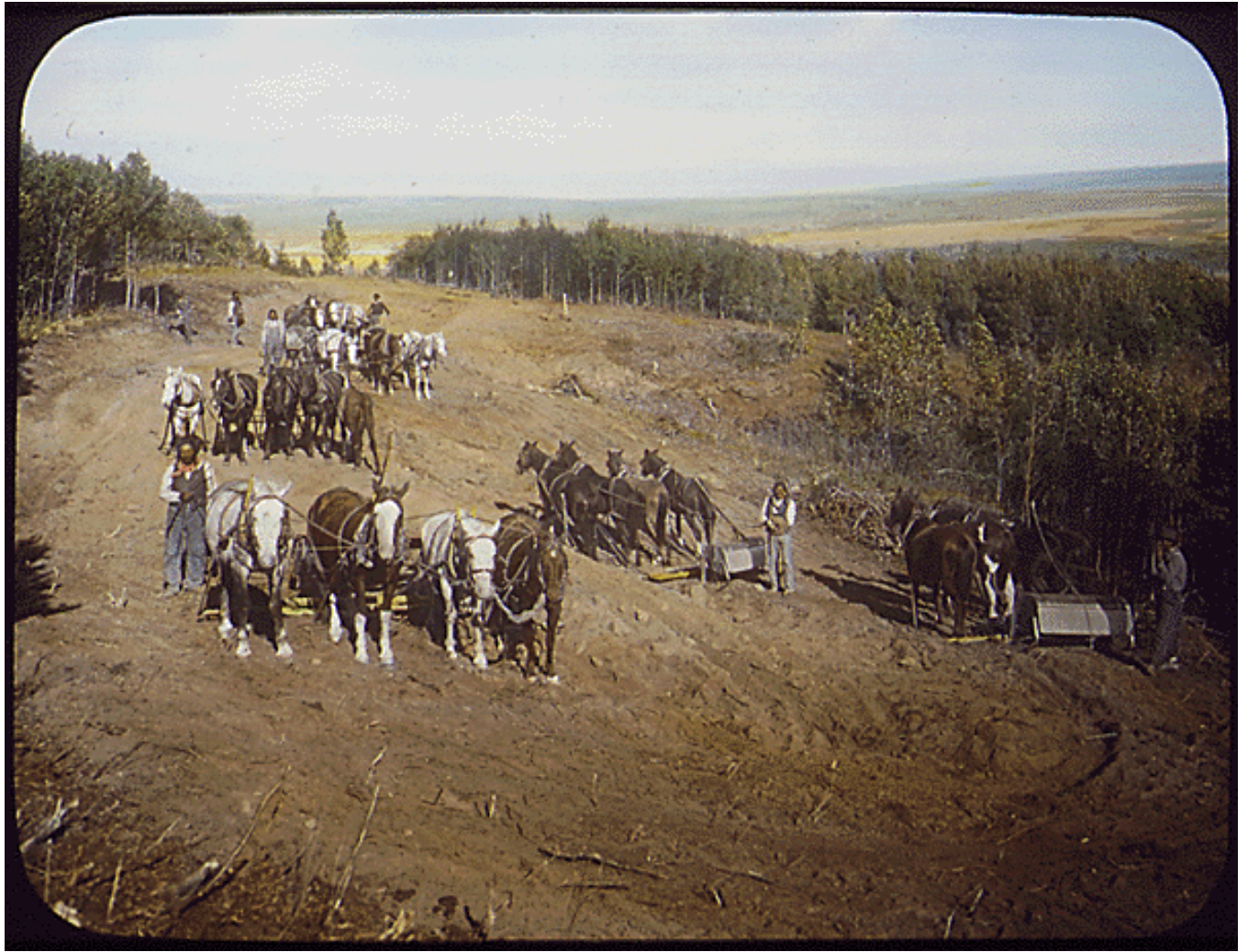
Site preparation work. Circa 1900s
