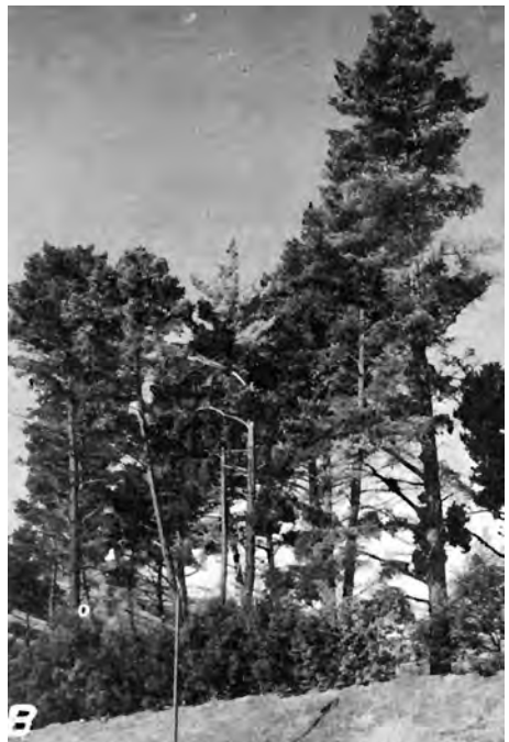
Figure 2.—Damage to Monterey pine by ips beetles: A, Group-killing in young plantation of pole-sized trees; B, fading tree crown (center) and scattered fading limbs in tree crown (right) in stand of mature trees.
