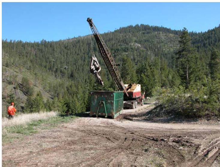
Figure 9. Loading roadside staged roll on/off container.
