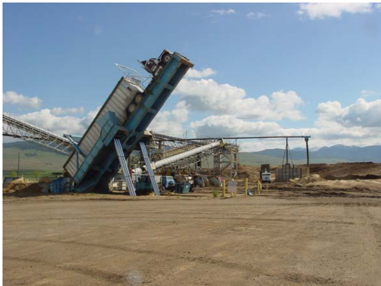
Figure 11. Unloading roll on/off container contents at Stimpson mill yard.
