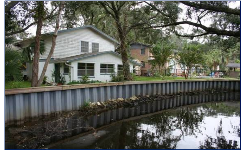
Floodwall in Jacksonville
