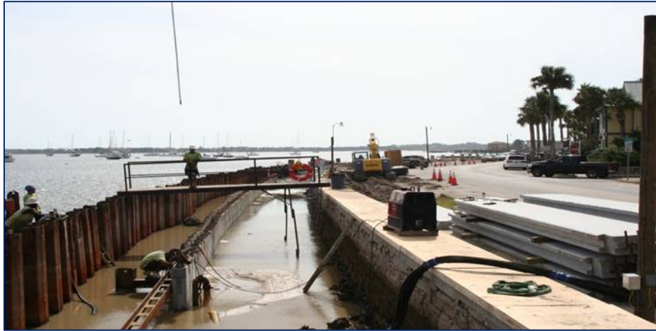
Seawall Construction in St. Augustine
